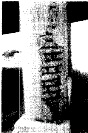
Corroded concrete column
