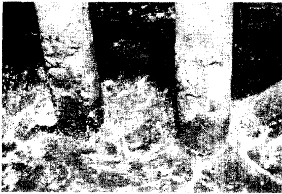
Corroded columns at water line
