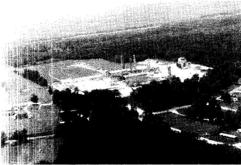
Gas distribution facility
