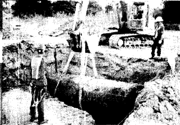
Lifting underground storage tank
