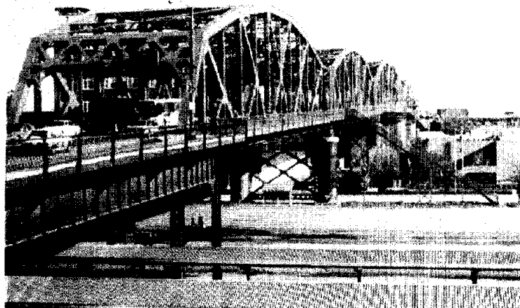
Figure 3. Steel bridge structure.
