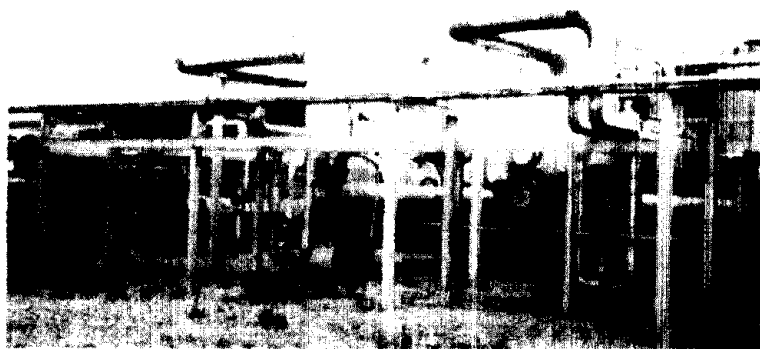
Figure 3. Typical plant piping in a petrochemical plant.
