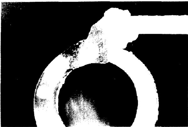
Cracked weld in stainless steel
