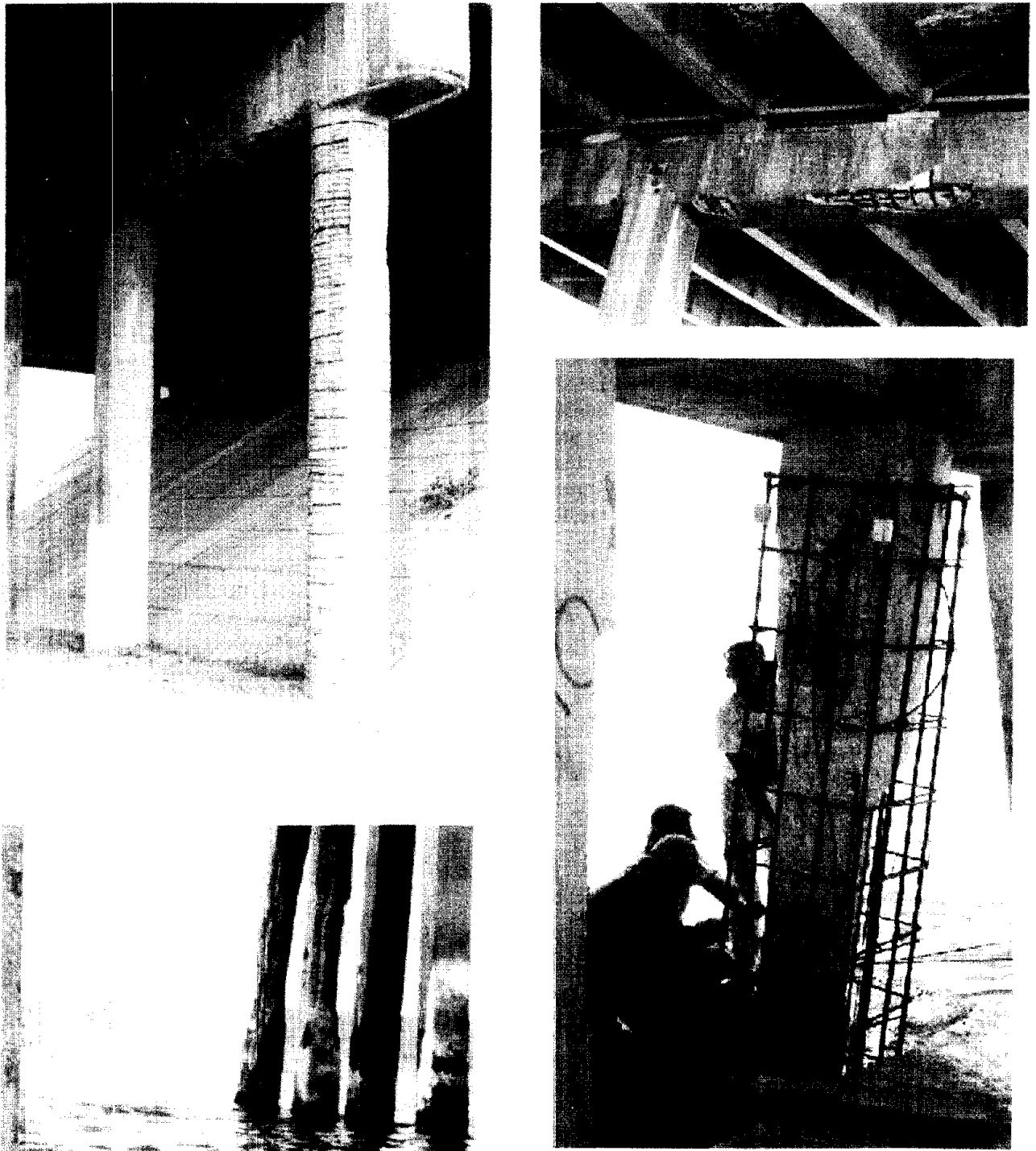
Figure 10. Examples of substructure corrosion.
