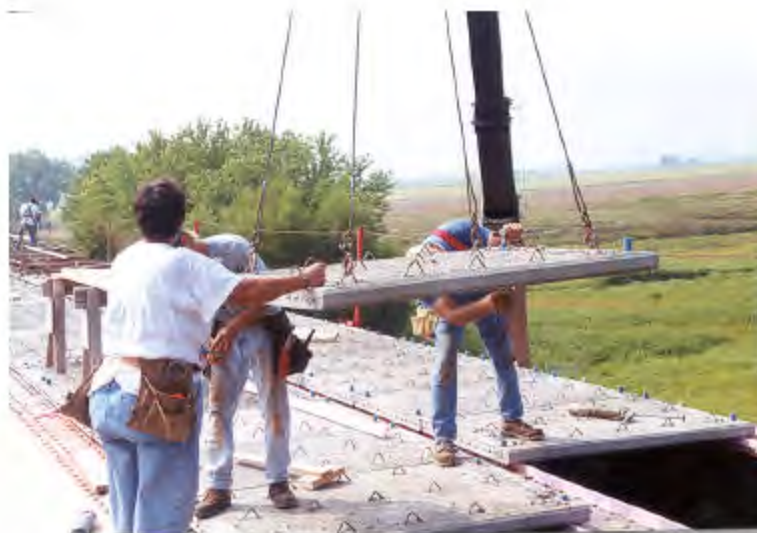
Photo 7. Deck plank seating (District 8 – Stage 2, Sept. 2, 1999)
