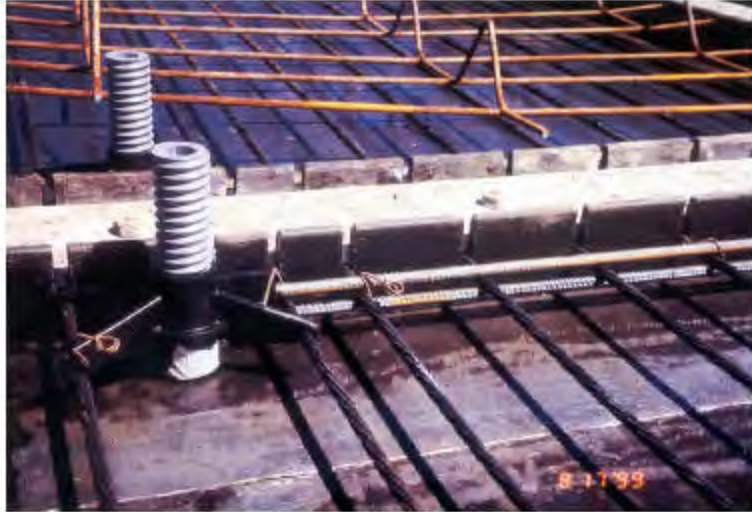
Photo 4. #3 rebar above and below strands
