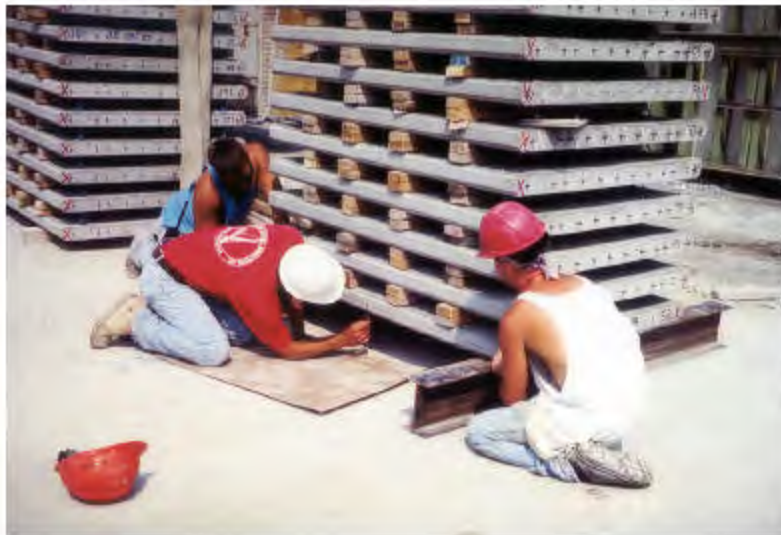
Photo 6. Checking deflection with stringline
