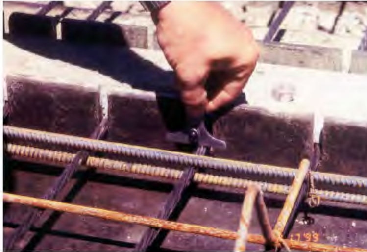
Photo 3. Checking vertical location of strand with micrometer
