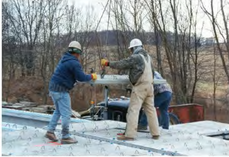
Photo 9. Deck plank seating (District 6 – Stage 2, Dec. 1, 1999)
