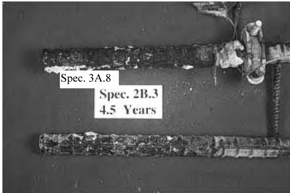
Figure 2.32 Corrosion at bottom side of cathodic, bottom bars of specimen 3A.8.
