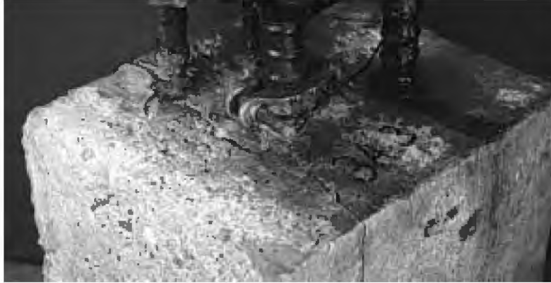
Figure 3.37 Severe concrete scaling on specimen 3A.8 with uncoated bars.
