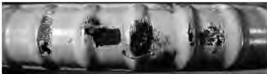
(a) Pitting corrosion on specimen 3B.3
