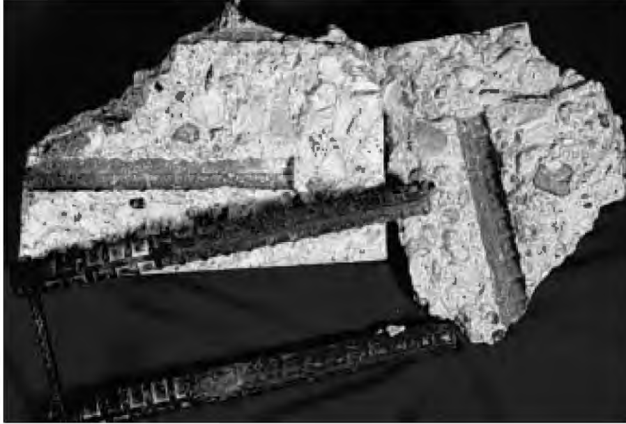
Figure 2.31 Cathodic uncoated bars at bottom of macrocell specimens.
