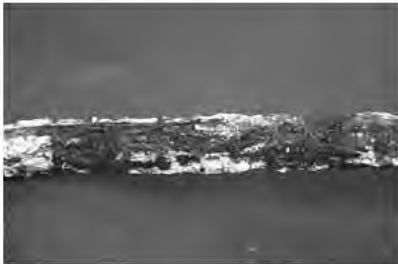
(b) Severe metal loss and pitting at straight leg of 13-mm (#4) uncoated bar after 4.5 years of exposure.
