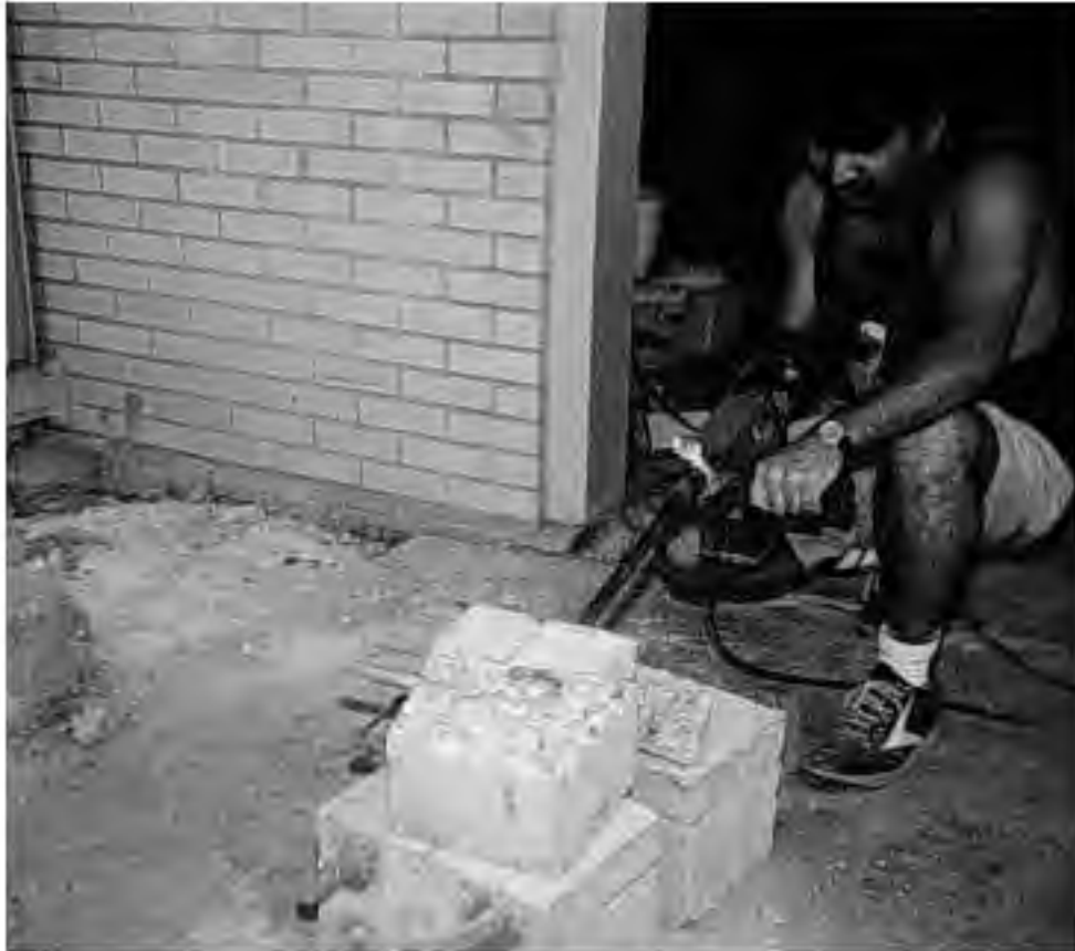
Figure A.27 Demolishing macrocell specimens.
