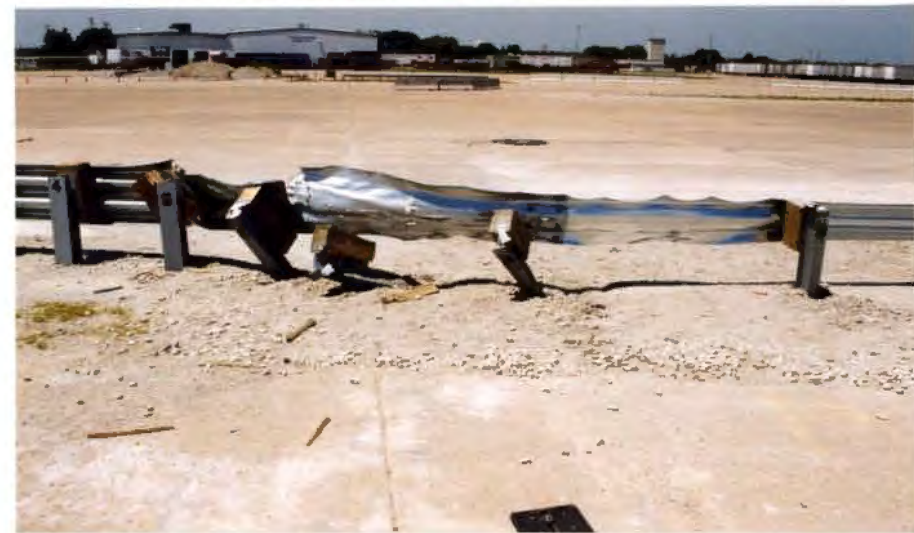
Figure 44. W-beam to Thrie Beam Transition Damage, Test MWT-2
