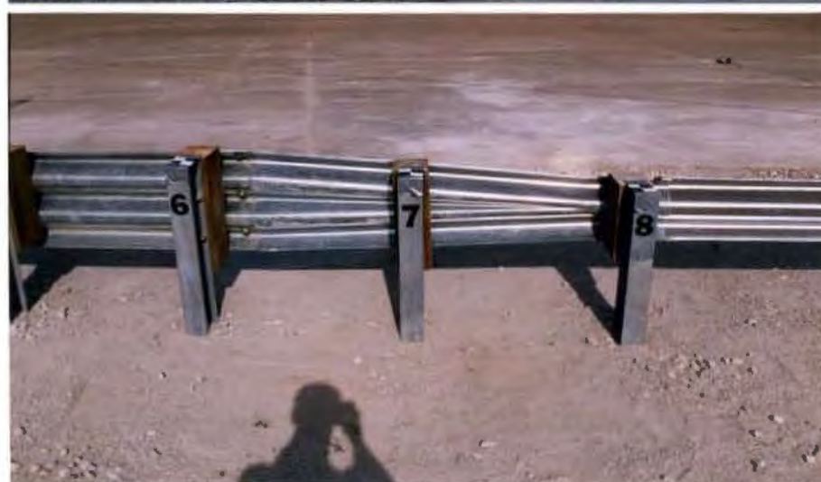
Figure 10. W-beam to Thrie Beam Transition (Continued)
