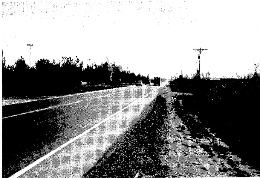
Figure 2. Looking south on Peger Road prior to installation of the surface treatments.
