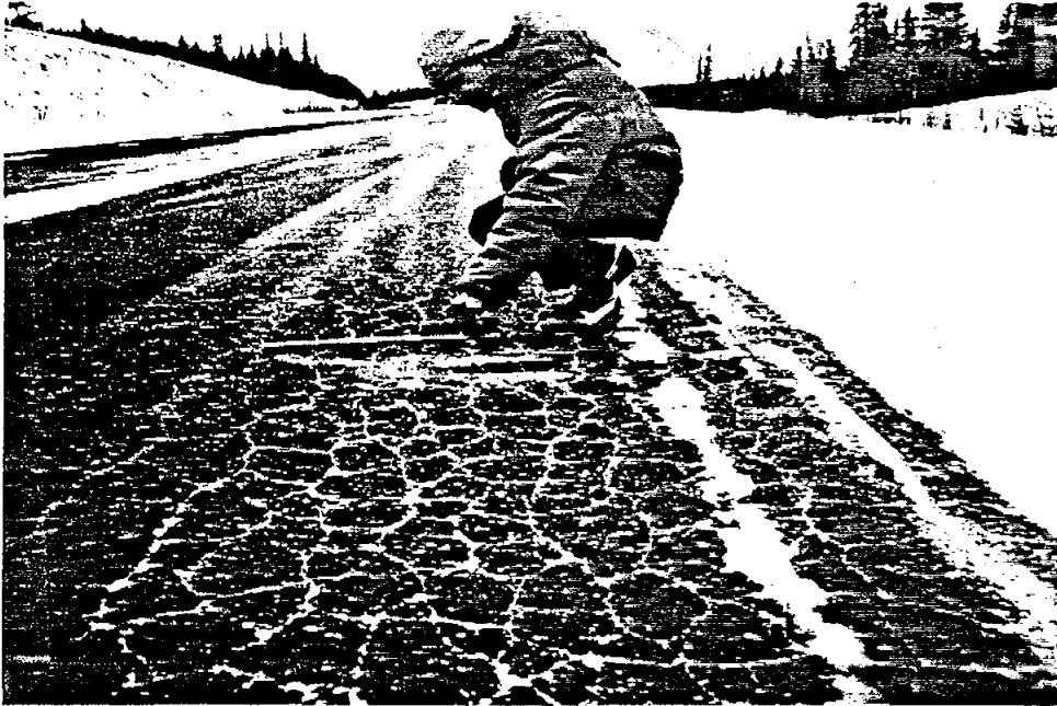
Figure 4.6 Permanent Deformation, Parks Highway.
