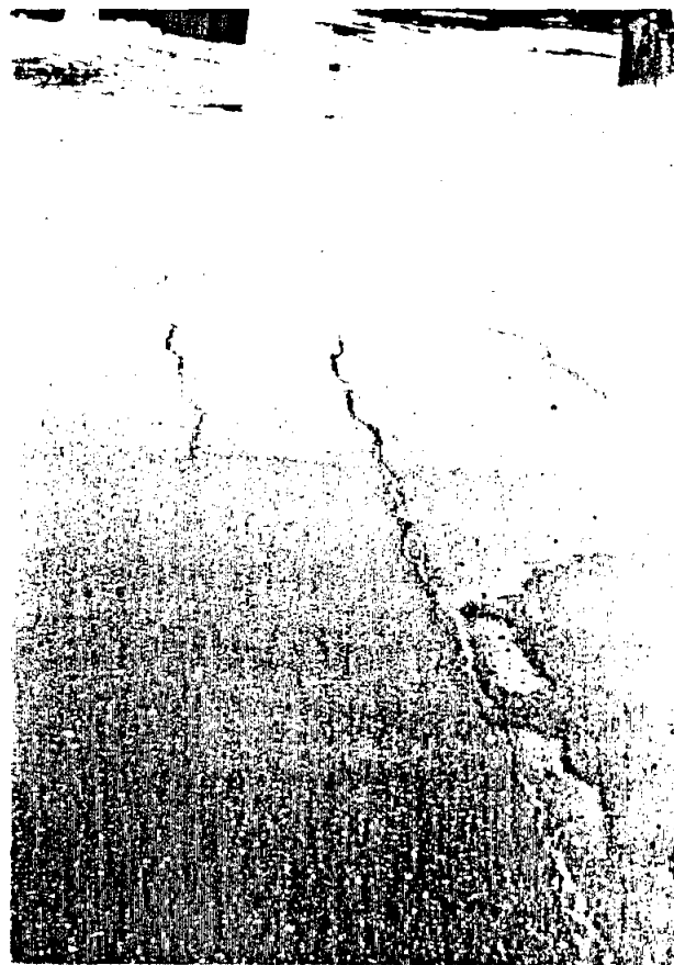
Figure 4.5 Pavement Surface Distress, Seward Highway.
