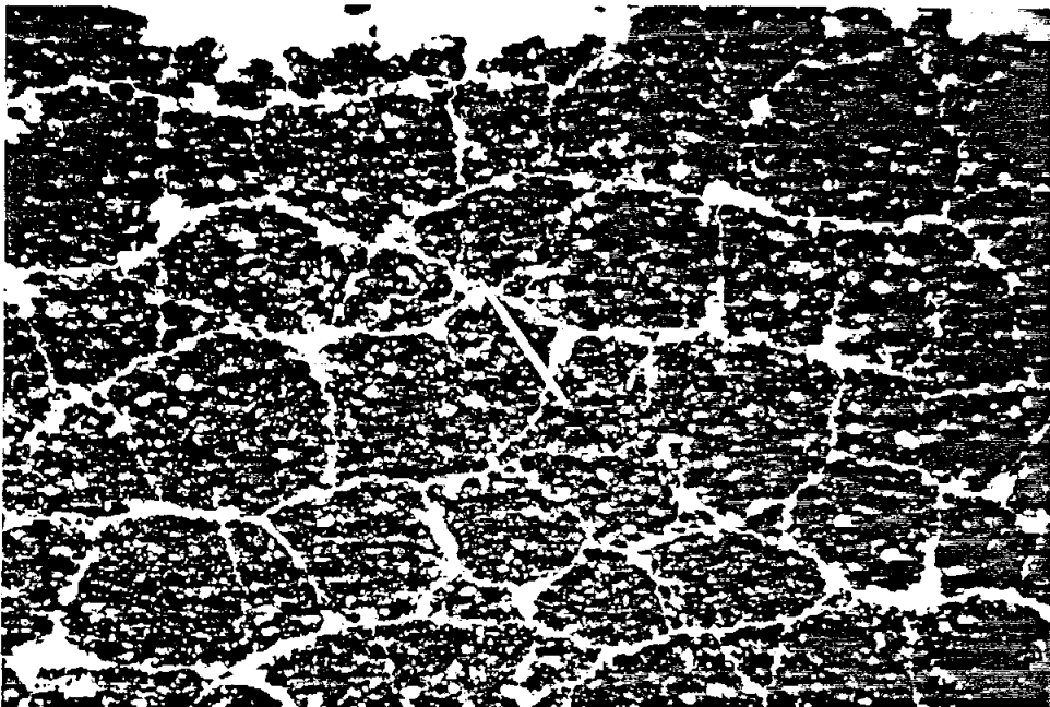
Figure 4.7 Alligator Cracking, Parks Highway.
