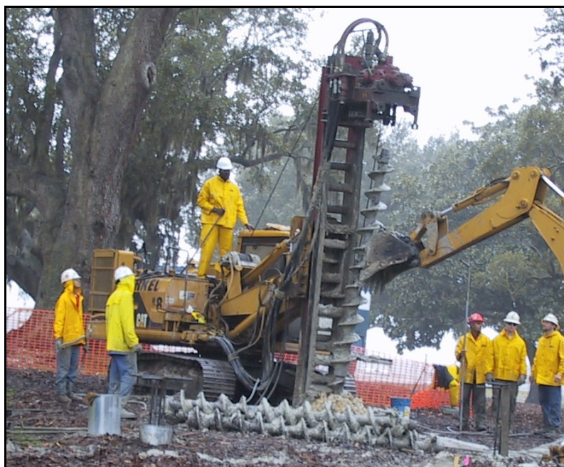
Figure 4.4: Low Headroom Rig with Segmental Augers
