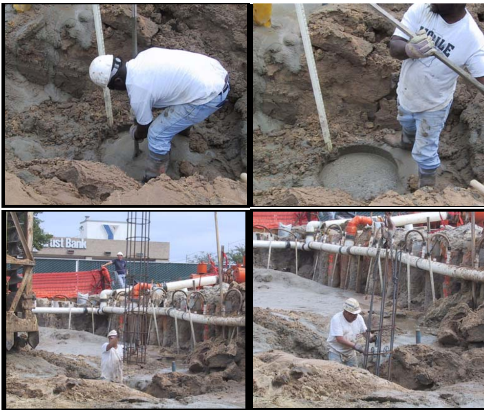
Figure 2.10: Finishing Pile and Reinforcement Placement
