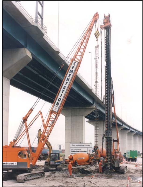
Figure 3.3: CFA Piles at Bridge Interchange
