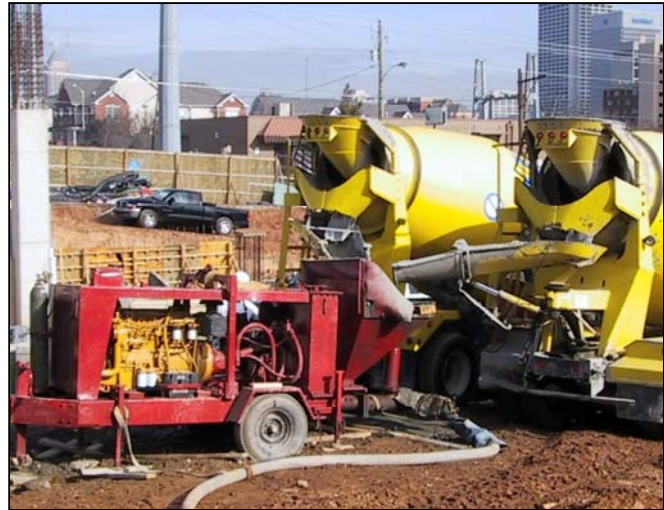
Figure 2.8: Grout Delivered to Pump
