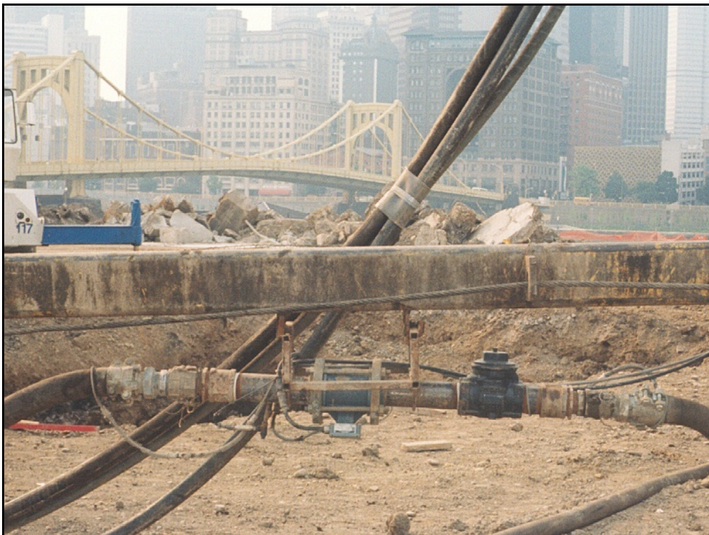
Figure 7.3: In-line Flowmeter
