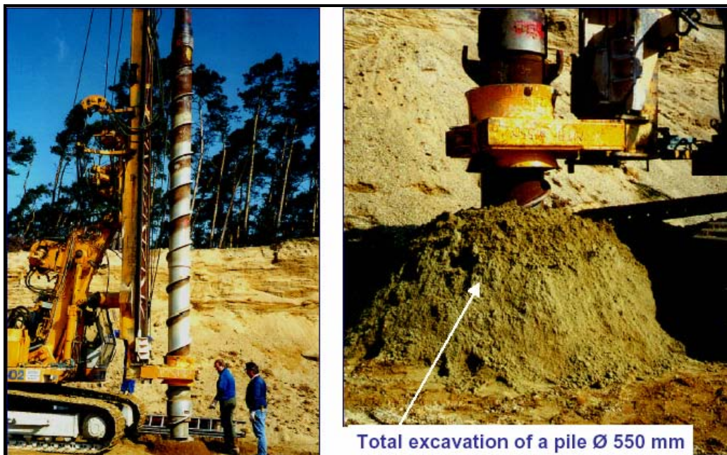
(b) Partial Displacement Auger
