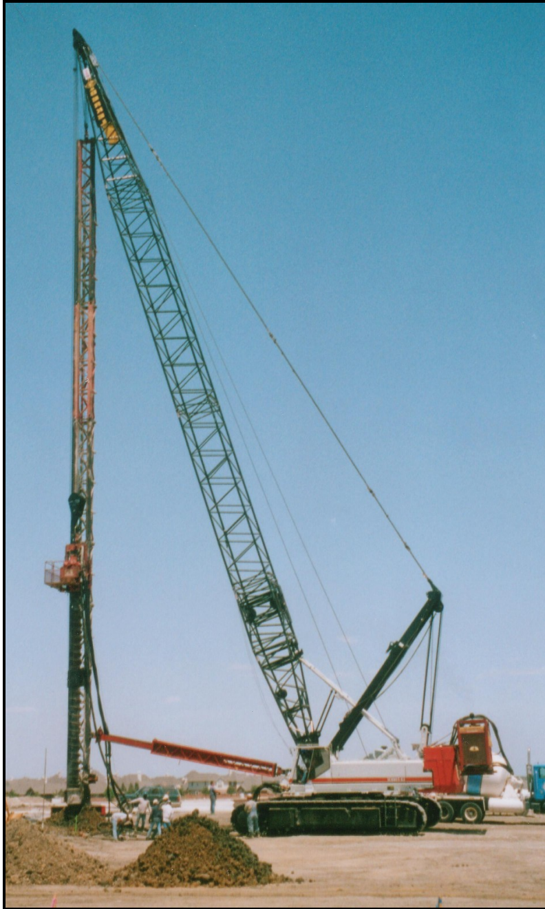
Figure 4.2: Photo of Crane-Attached CFA System
