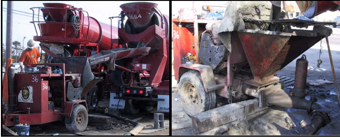
(a) Trucks Discharging into Pump
