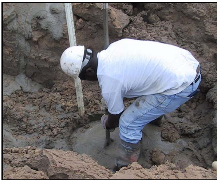
Figure 7.7: Dipping Grout to Remove Contamination
