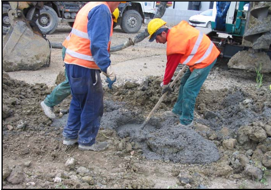
Figure 7.8: Cleaning the Top of a CFA Concrete Pile
