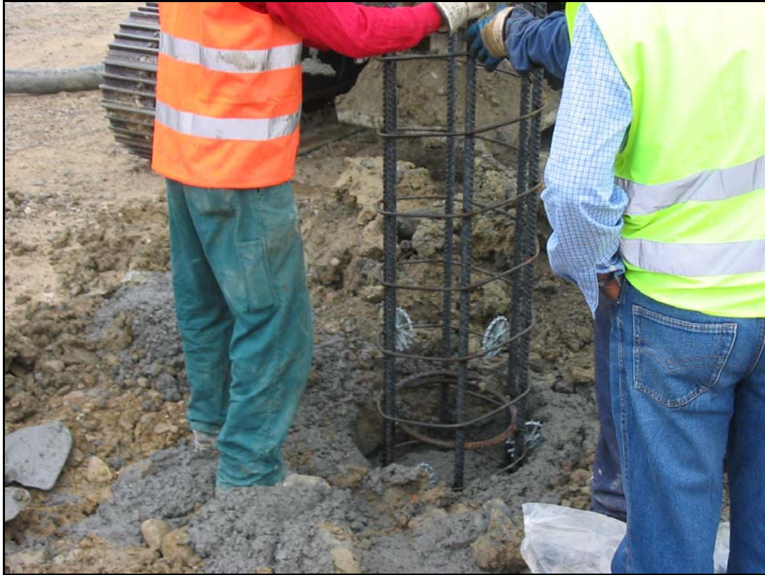
Figure 7.9: Placement of Reinforcing Cage with Plastic Spacers
