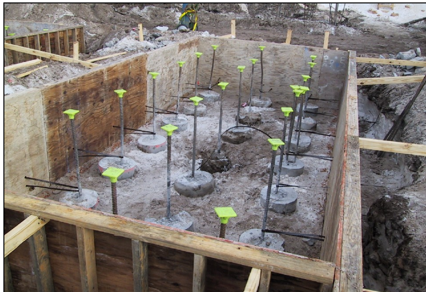
Figure 2.4: Group of CFA Piles with Form for Pile Cap
