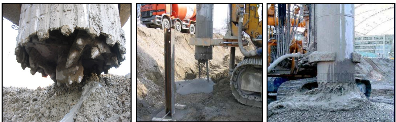
(a) Cutting Head (b) Concrete Placement (c) Cuttings Discharge
