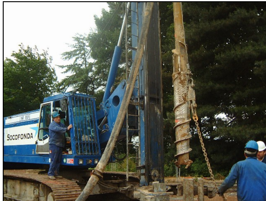
Figure 4.12: Omega Screw Pile
