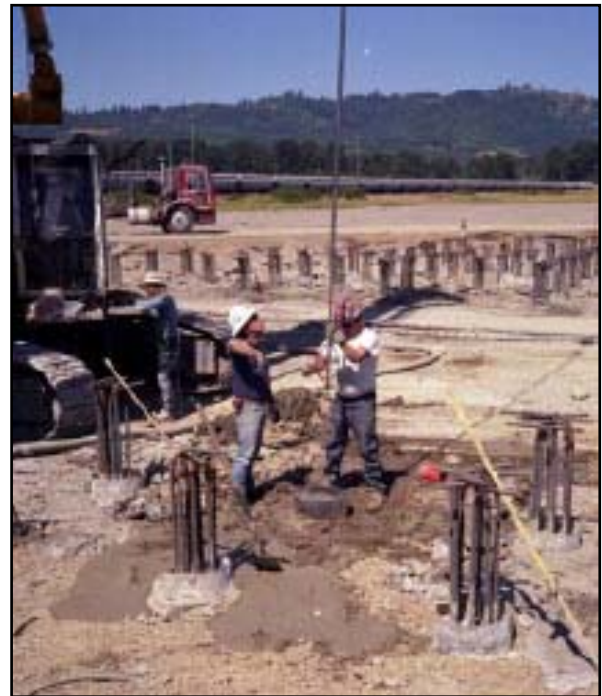
Figure 2.11: Placement of a Single Full-Length Bar
