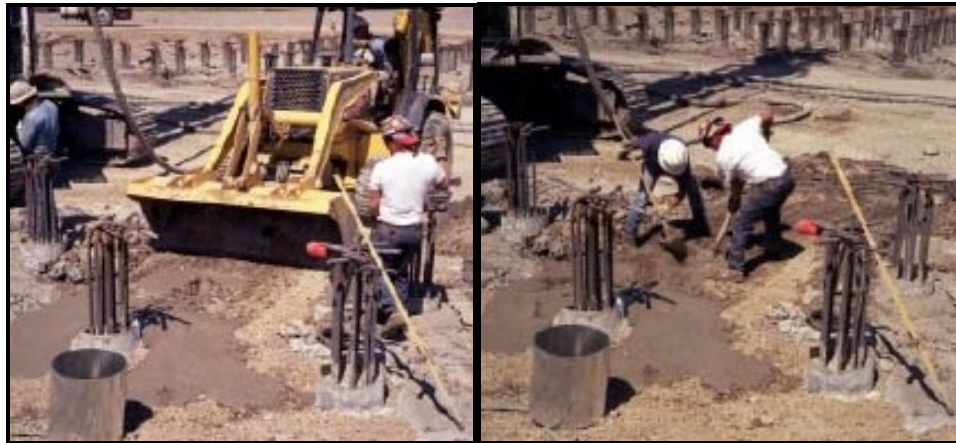
(a) Spoil Removal
