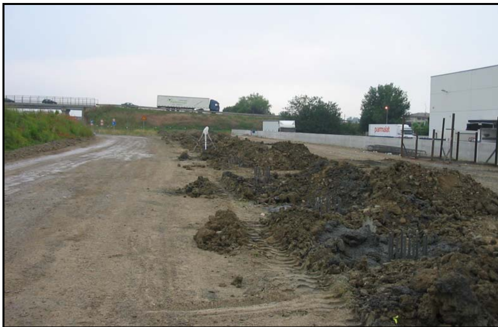
Figure 3.6: CFA Piles for Soundwall (at right) along Highway (out of view to left)
