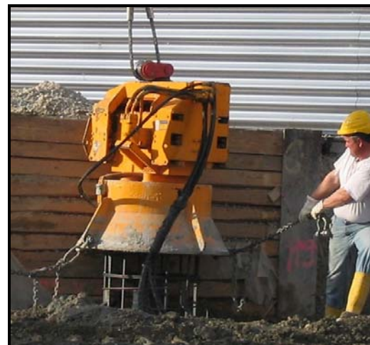
Figure 2.12: Vibratory Drive Head Used to Install Rebar Cage
