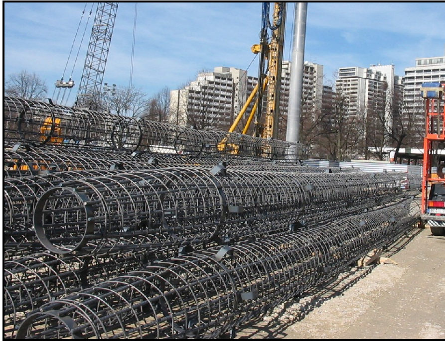
Figure 4.24: Machine-Welded Reinforcement Cage on Project Site in Germany
