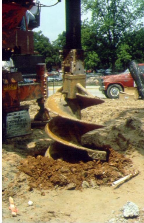
Figure 3. Large diameter auger boring.
