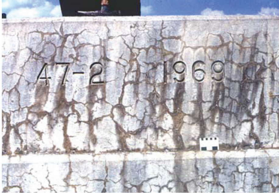
Figure 5 – Gel Exudation (Condition State 3)
