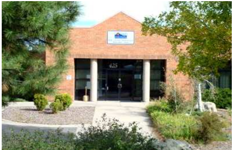
Exhibit A5 – New CTMC Building Entrance
