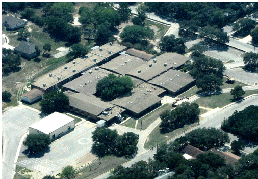
Figure 17: Aerial View of Old Crockett
