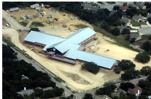
Figure 19: Aerial View of New Crockett Site
