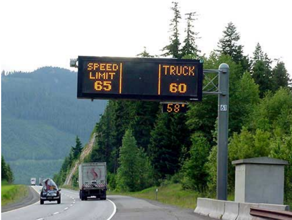
Figure 1.1: Variable Speed Limit System on I 90 at Snoqualmie Pass (Source: Washing State DOT, 2006)
