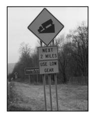
Use of too many supports, either on one sign or for a group of signs can produce a hazard. This supporting system is too rigid and may contribute to overturning, loss of control or abrupt stopping.
