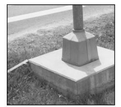
While the system used is a break-away base the pedestal it is mounted on was either not back filled around or the soil has eroded around it. This support system is now a hazard as it constitutes a rigid concrete block more than four inches above the surrounding ground. This can snag the under-carriage of a vehicle causing it to stop abruptly or go out of control.
