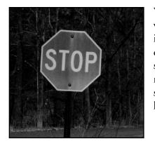
When a sign face becomes so worn or faded that the message is not legible or can be misread during daytime or night, the sign should be replaced. A sign needs to be readable in ordinary sunlight and still reflect enough light at night to be a useful sign.
