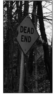
Signs may be bent like this DEAD END sign. While many bent signs can be read in the daylight, some bent signs, even signs with minor bending, are difficult to see at night because they no longer reflect the light from the vehicle's headlights back to the driver's eyes. Minor bending like this may be repaired by removing the sign from the post and straightening the sign face.
