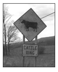
This sign is old and and the surface is seriously cracked – it has lost its retrorefflective characteristic and appears as a distorted image at night. If the signs are still appropriate they should be scheduled for replacement.
