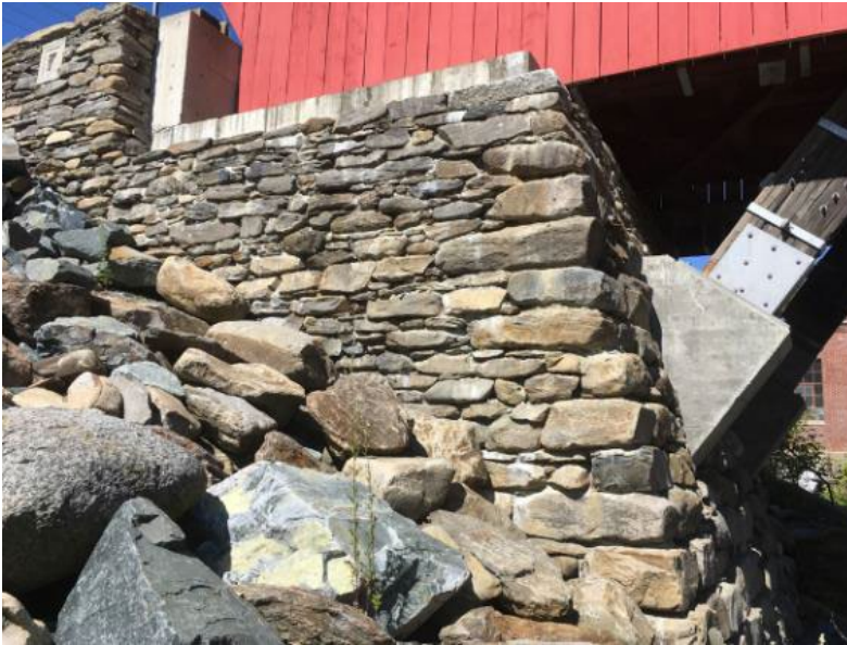
Figure 18: Southern Abutment and closeup of mortar leachate (2017)
