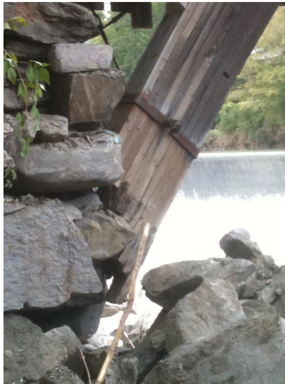
Figure 11: Downstream western arch dislodged from abutment
