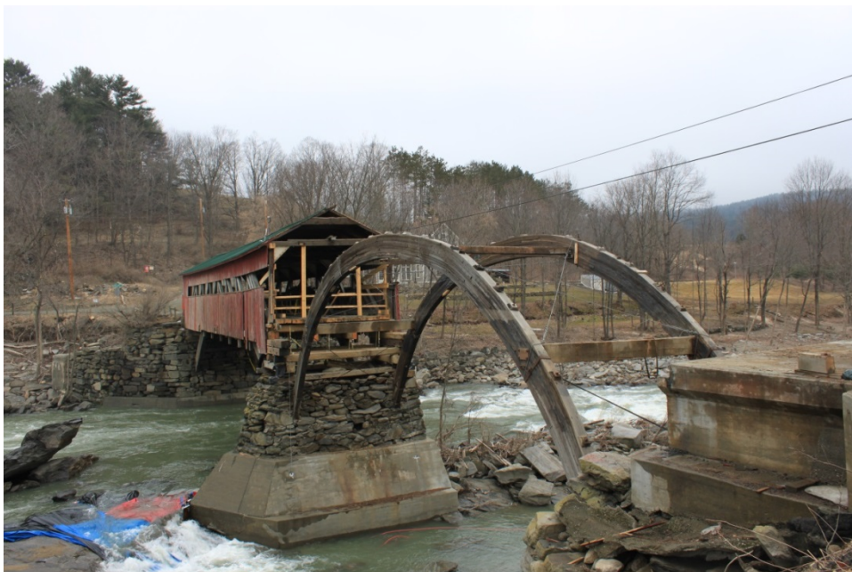
Figure 10: Western span dismantled leaving only the arches
