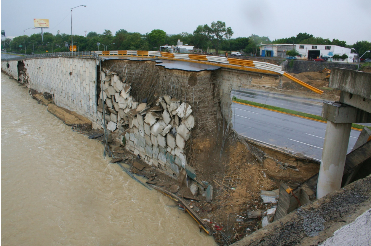
Figure 1-2. Metallic reinforced wall: limit state shallow failure [June 2010, Monterrey, Mexico, Hurricane Alex]
