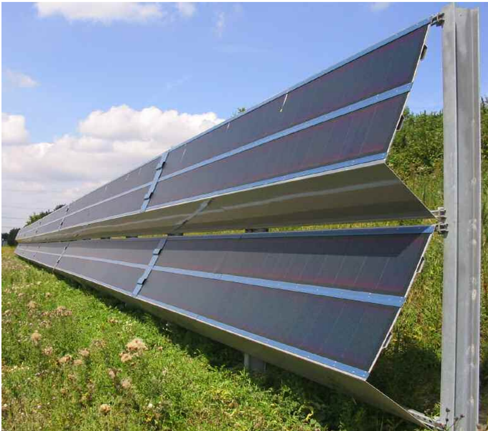
Figure 8. Completed installation of the solar laminates at the bottom of the slope
