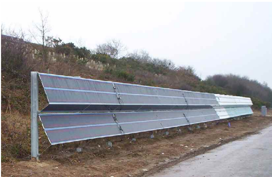
Figure 7. Installation of the solar laminates at the bottom of the slope
