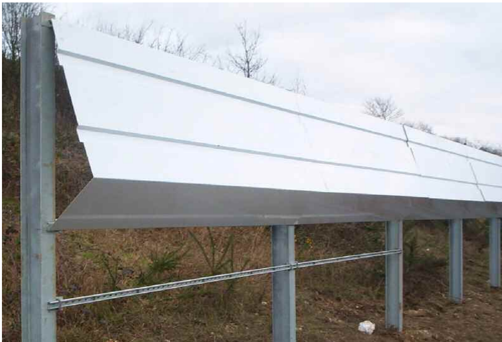
Figure 5. Installation of the folded sheet mountings
