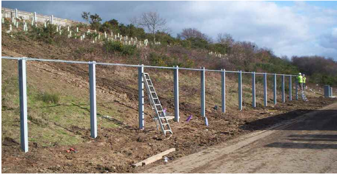
Figure 4. Installation of the galvanised steel posts
