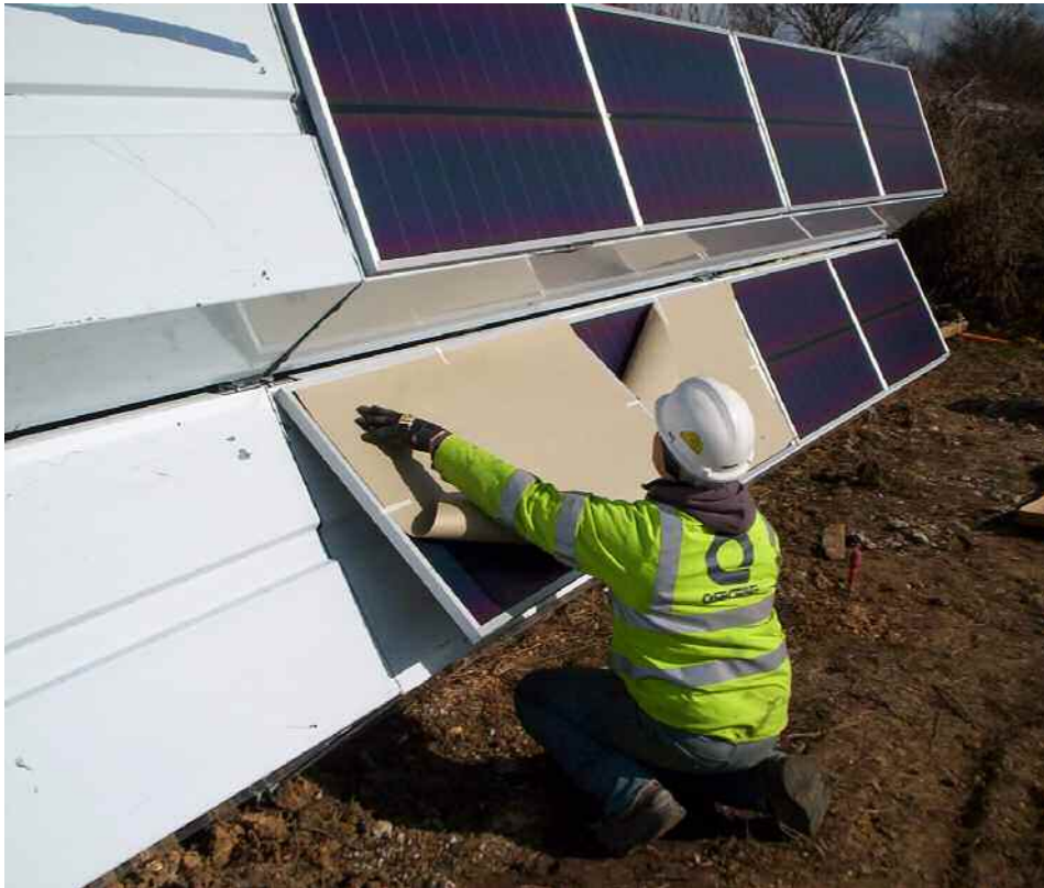
Figure 6. Installation of the solar modules at the top of the slope
