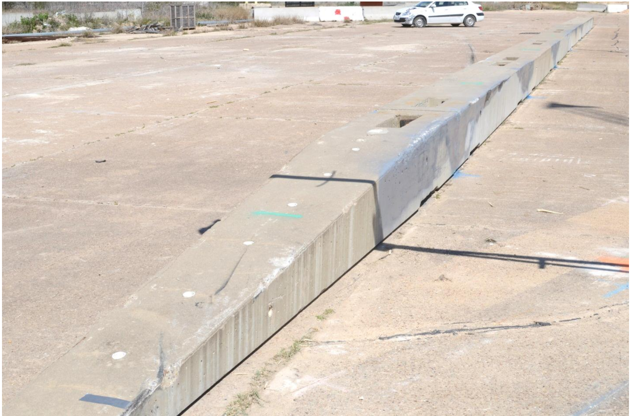
Figure 6.4. Installation after Test No. 490023-5.
