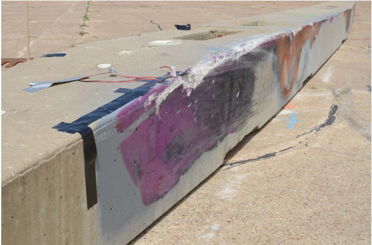
Figure 5.4. Installation after Test No. 490023-7.
