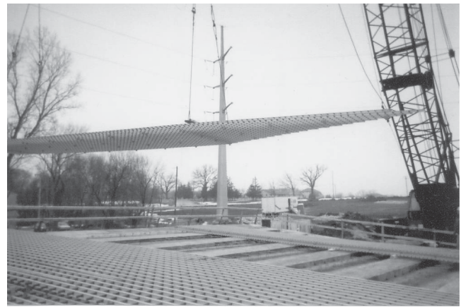
FIGURE 2 Installation of full-width double-layer grid.
