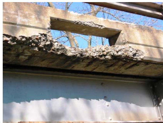
Figure 1 – Degradation of concrete deck, steel girders (a) and safety appurtenance (b) on Bridge 14802301, Greene County, MO
