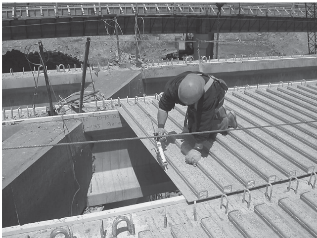
FIGURE 1 Installation of CDS deck panels.
