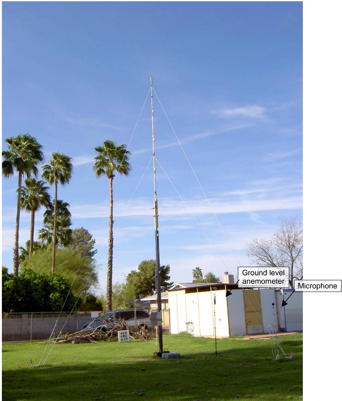
Figure 56. Meteorological Tower at Site 2 (8701 W. Highland Ave.), Looking Southwest
