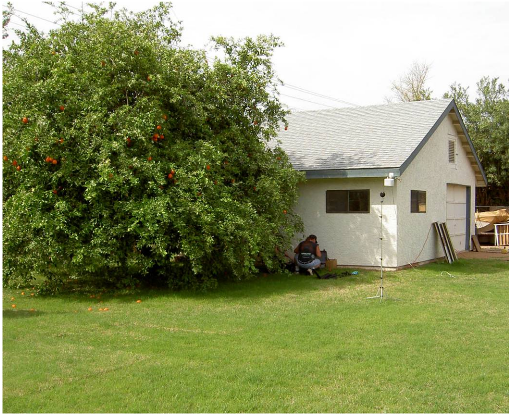
Figure 60. Site 3 (8547 E. Highland Avenue) Looking Southwest
