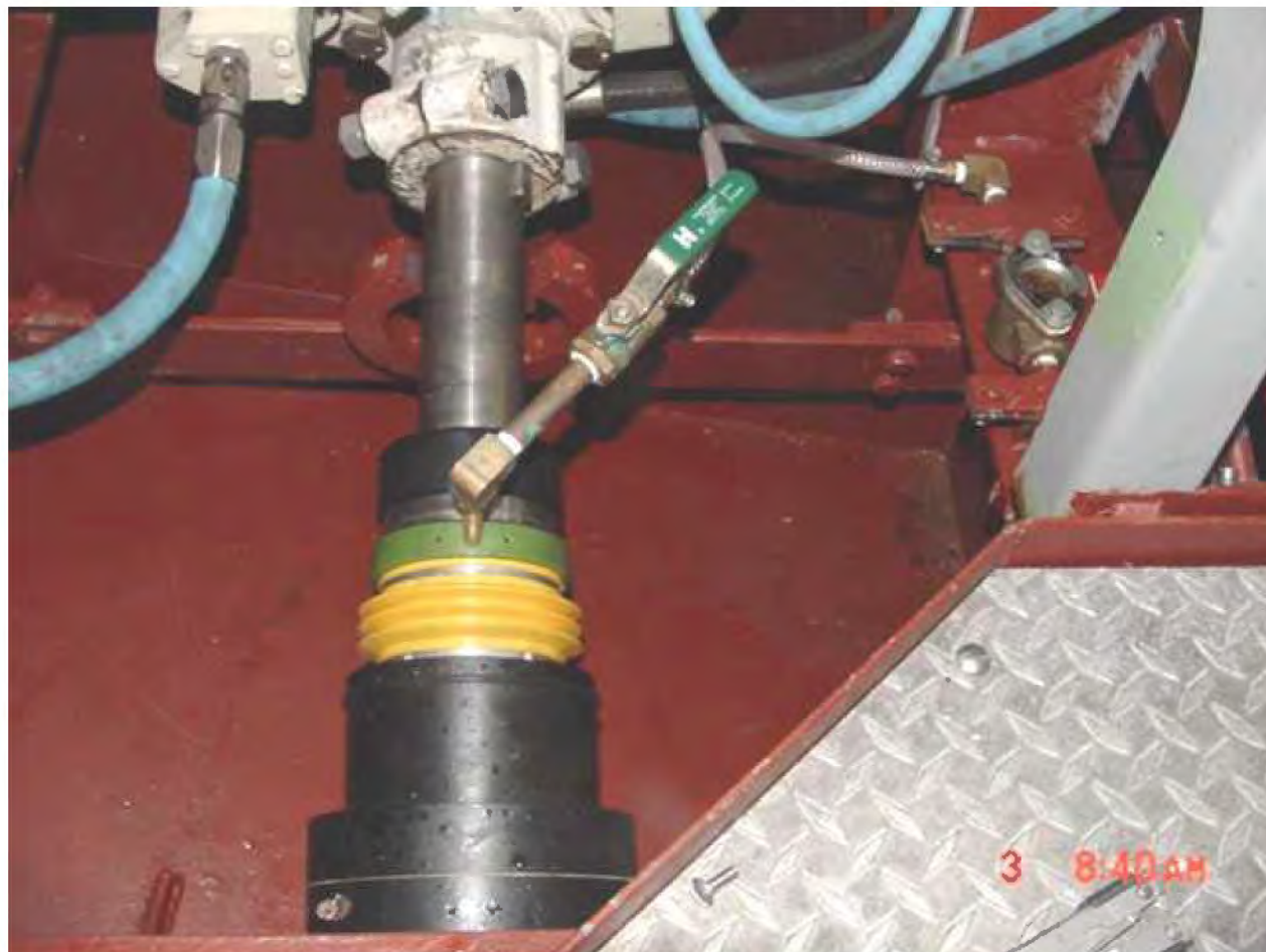
Figure 3-2 Shaft Seal Assembly
