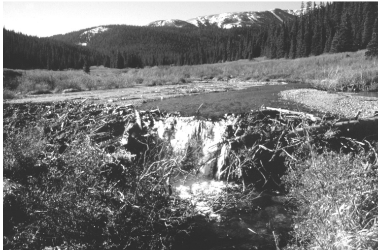
Figure 41. Abandoned beaver pond filled with sediment on South Clear Creek upstream from Lower Cabin Creek Reservoir, June 1996.
