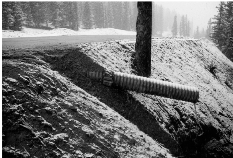
Figure 35. Culvert outflow concentrating road runoff onto the fillslope in the switchback road segment above South Clear Creek, upstream from Naylor Creek, July 1995.
