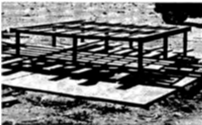
FIGURE 4. CONSTRUCTION OF TEST STANDS
