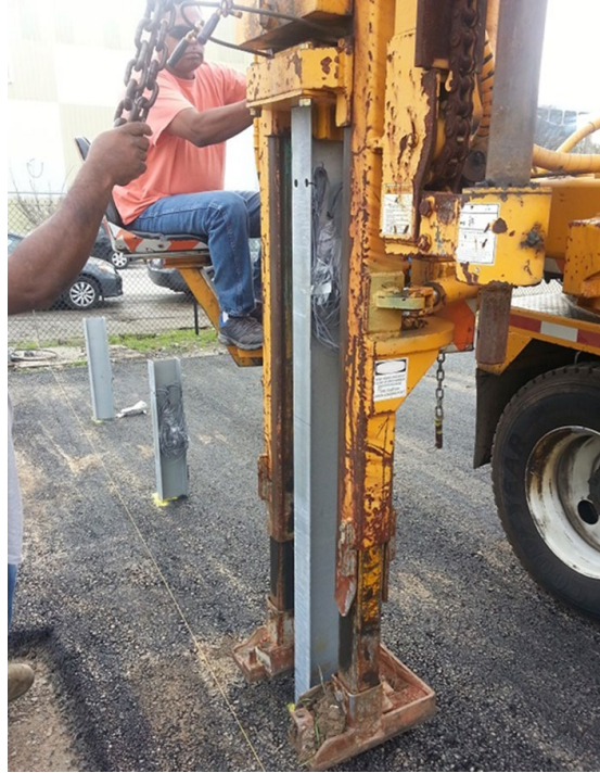
FIGURE 5 Typical Post Installation Procedure in Georgia
