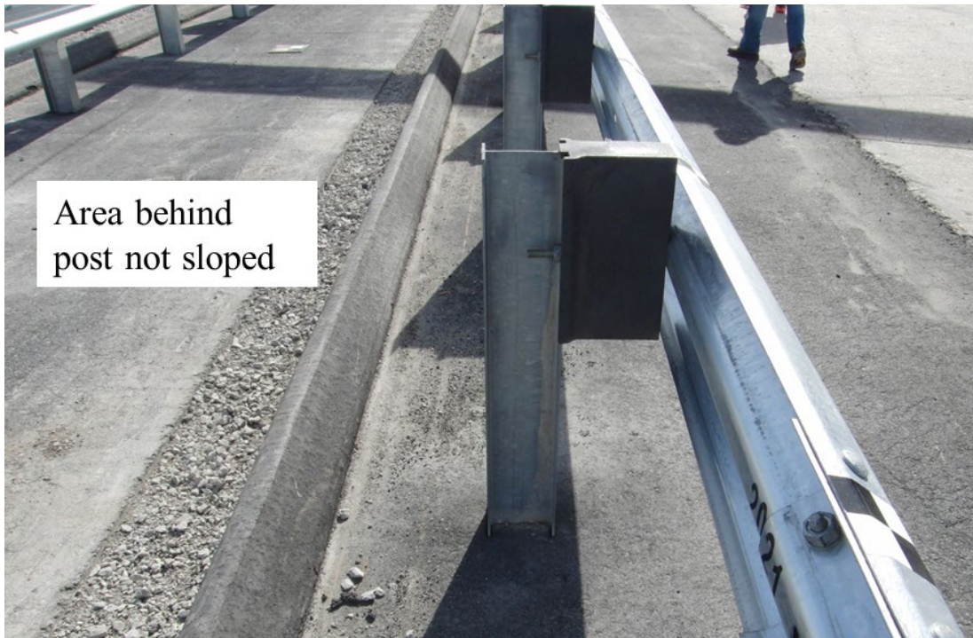
FIGURE 4 Test Bed Site – View Showing Area Directly Behind the Post
