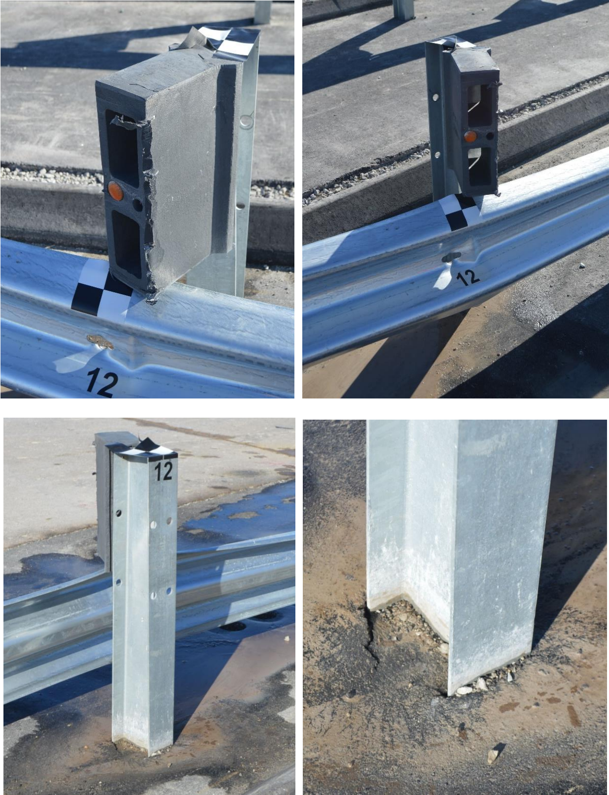
Figure 40. Post No. 12 Damage, Test No. GAA-1
