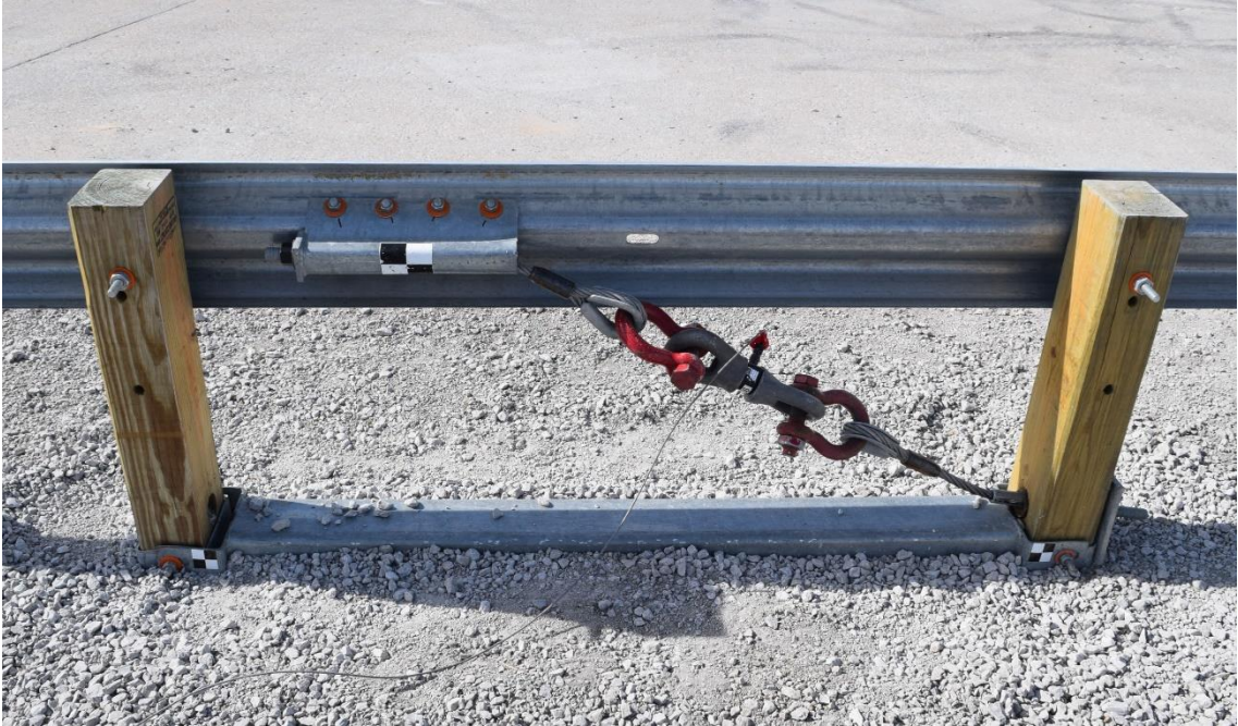
Figure 27. Location of Load Cell (Downstream Anchorage)
