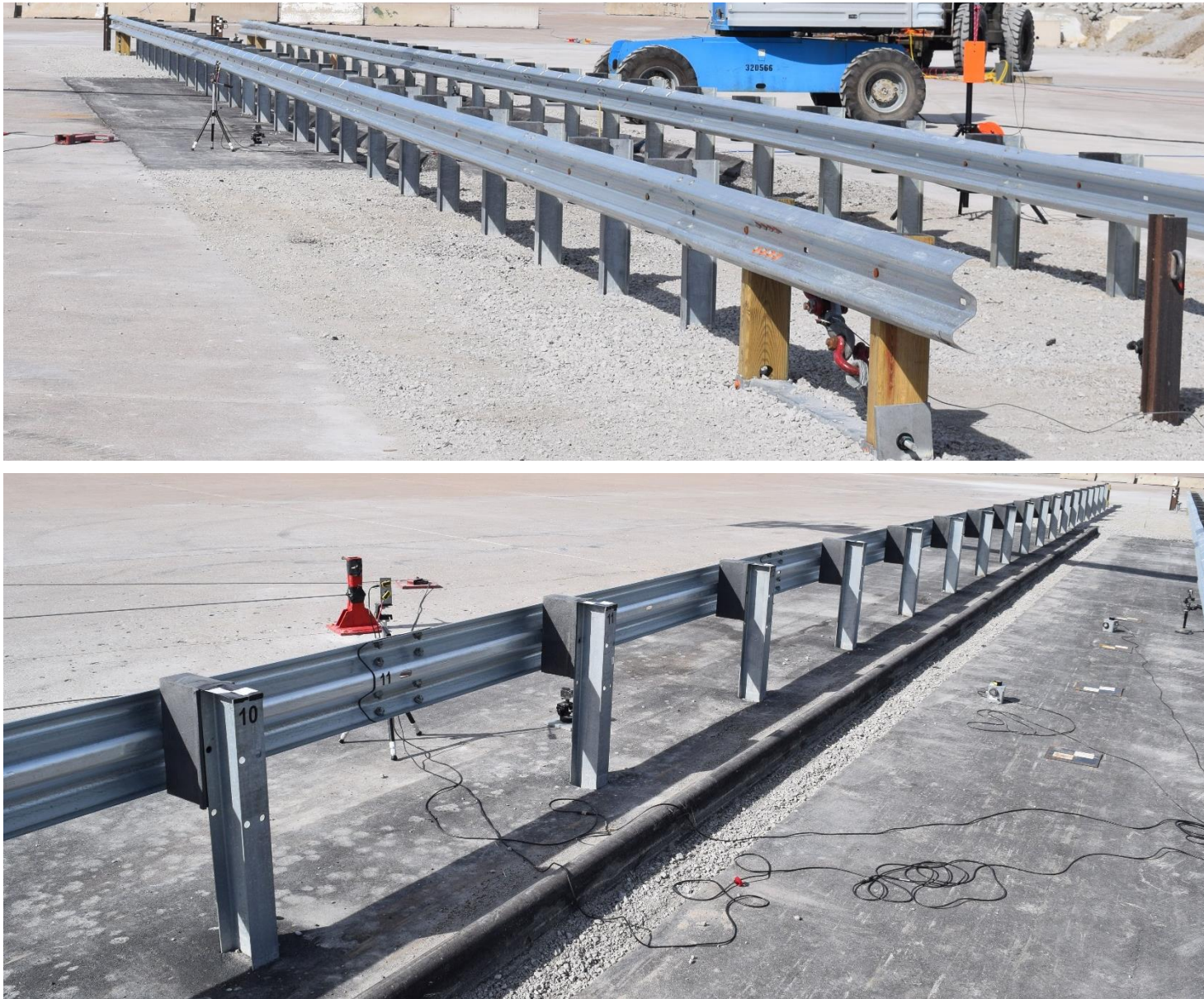
Figure 20. Test Installation, Test No. GAA-1
