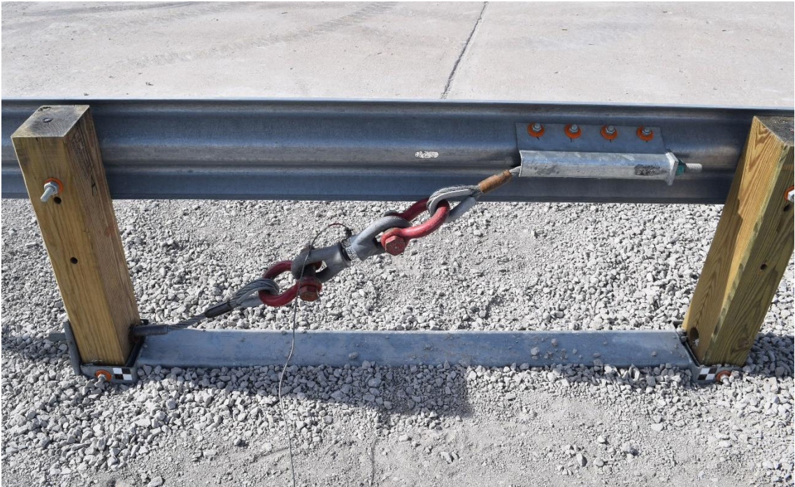
Figure 28. Location of Load Cell (Upstream Anchorage)
