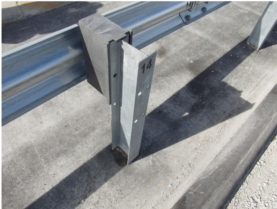
FIGURE 6 Typical Post Installation at MwRSF Test Site
