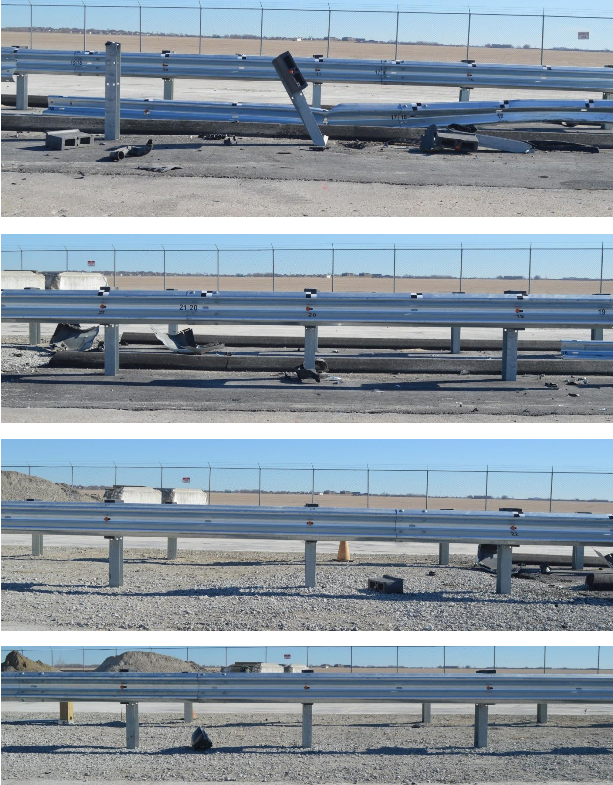
Figure 39. System Damage – Post Nos. 16 through 27, Test No. GAA-1
