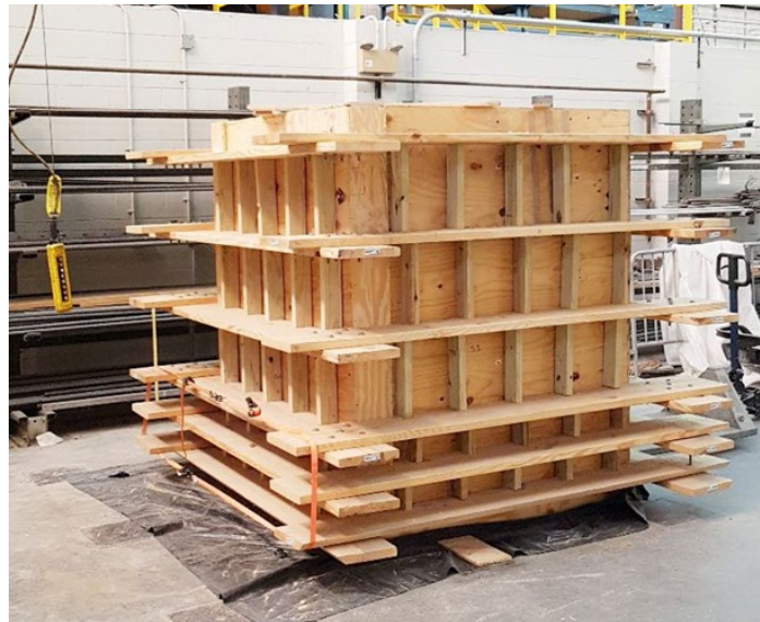
Figure 9. The concrete form for the mid-scale specimen
