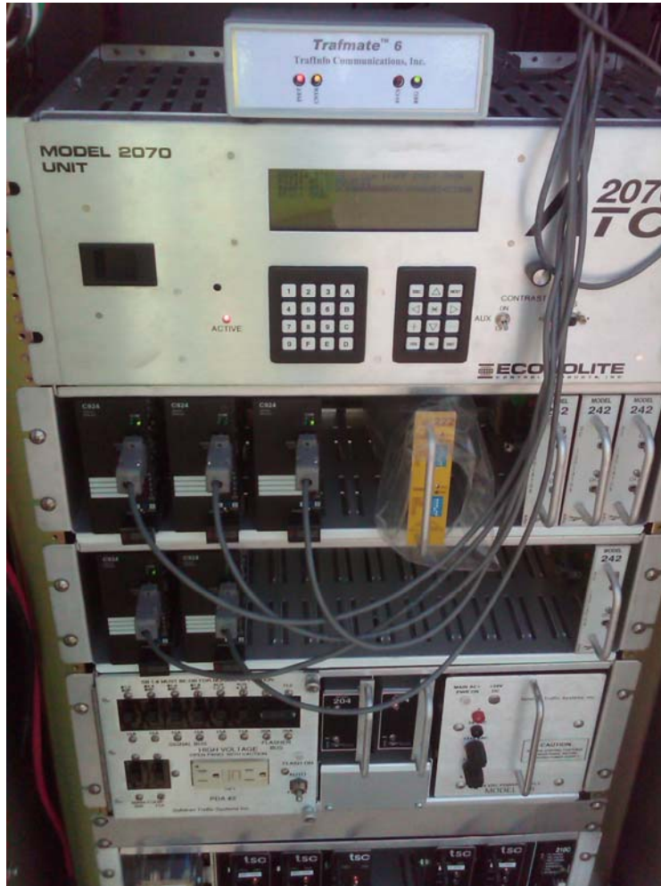
Figure 3. TrafMate 6 Device (top) and Five Canoga Cards (mid-left). (Courtesy Sudhir Murthy, TraffInfo Communications, Inc.)
