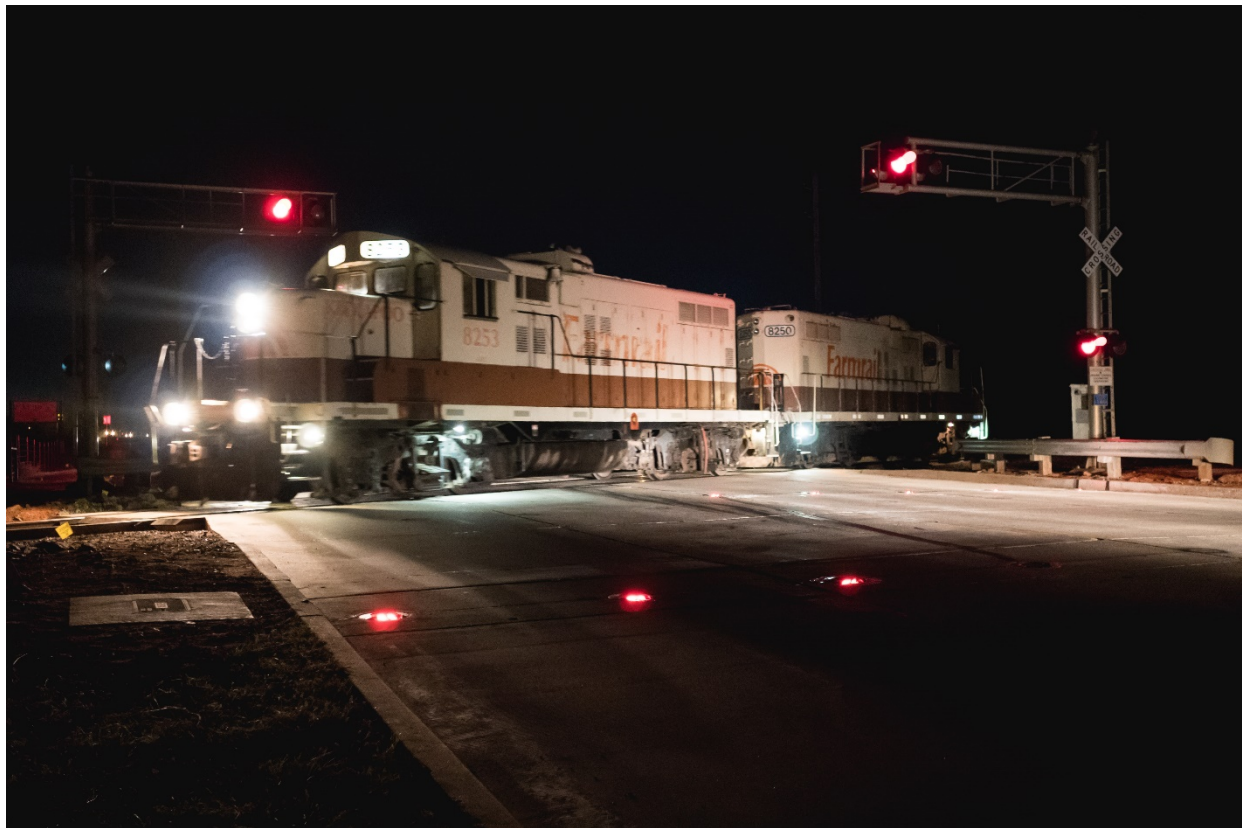
Figure 3 – Elk City in-pavement lights, looking west
