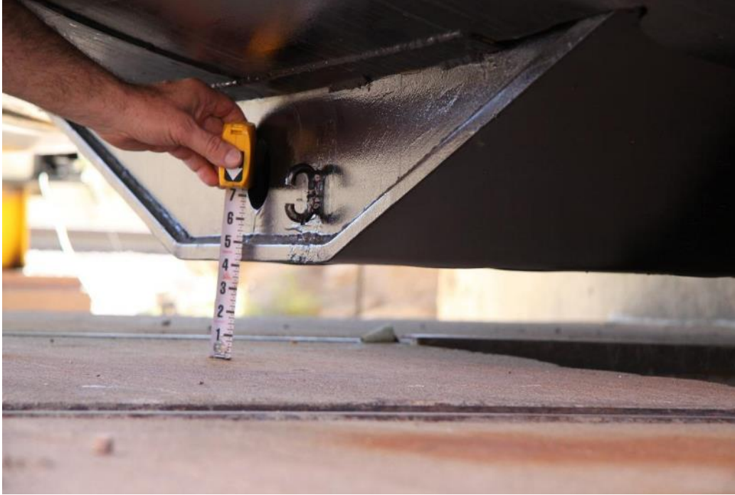
Figure 31. Pre-Test Vertical Clearance of Bottom Protection (Photo Courtesy of Kathi Kube)
