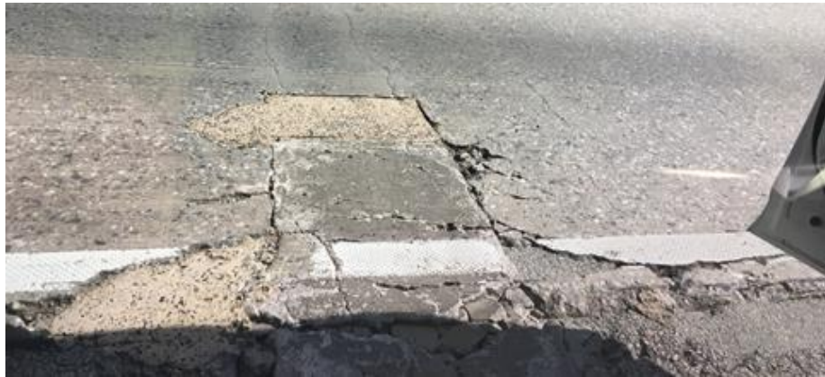
Figure 2-2 Severity Level 2 punchout
