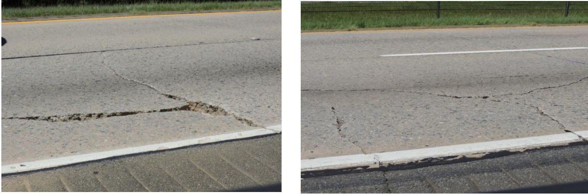
Figure 4-3 Examples of shattered slab
