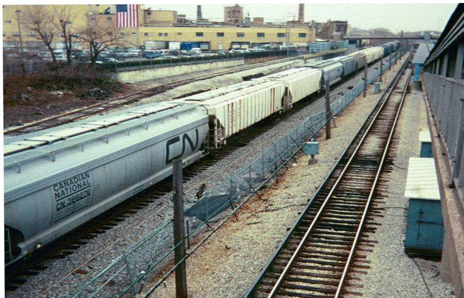
Figure 16: View of CSX trackage and freight train at Laramie Ave., Blue Line
