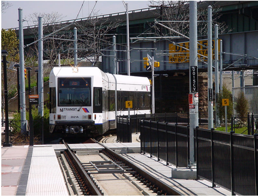
Figure 29: HBLRT Train at Liberty State Park station
