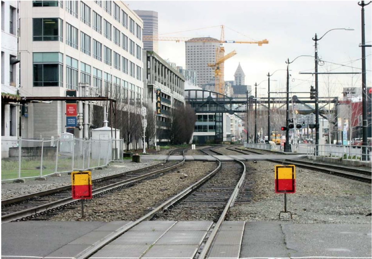
Figure 77: Looking South Toward Downtown, BNSF Tracks to Left, Streetcar to Right
