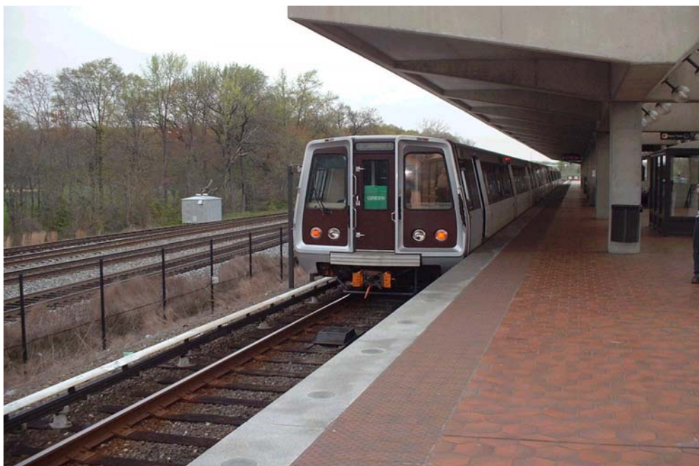
Figure 84: Metro train at Greenbelt
