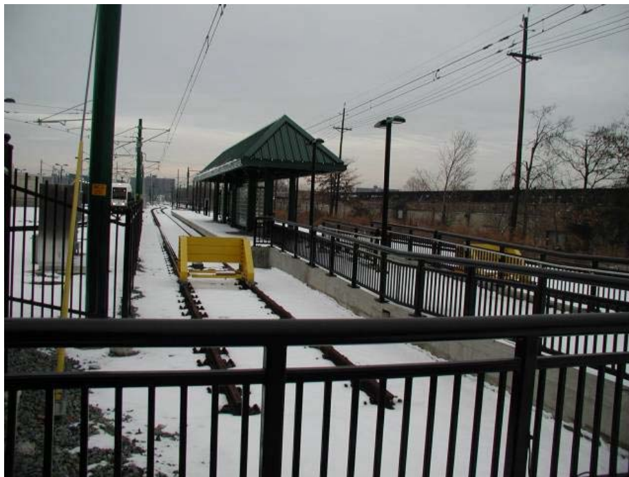
Figure 39: Grove Street Station
