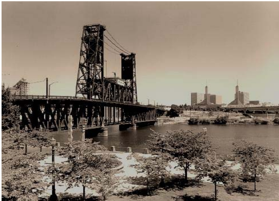
Figure 55: Steel Bridge, Portland, OR
