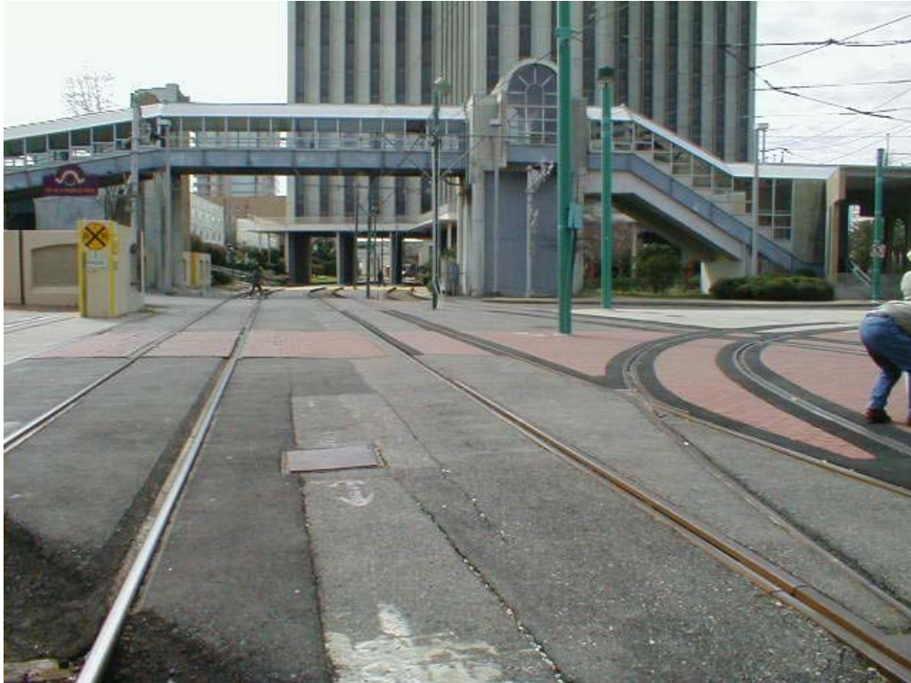
Figure 40: Junction of Canal and Riverfront Lines, NOPB track to left
