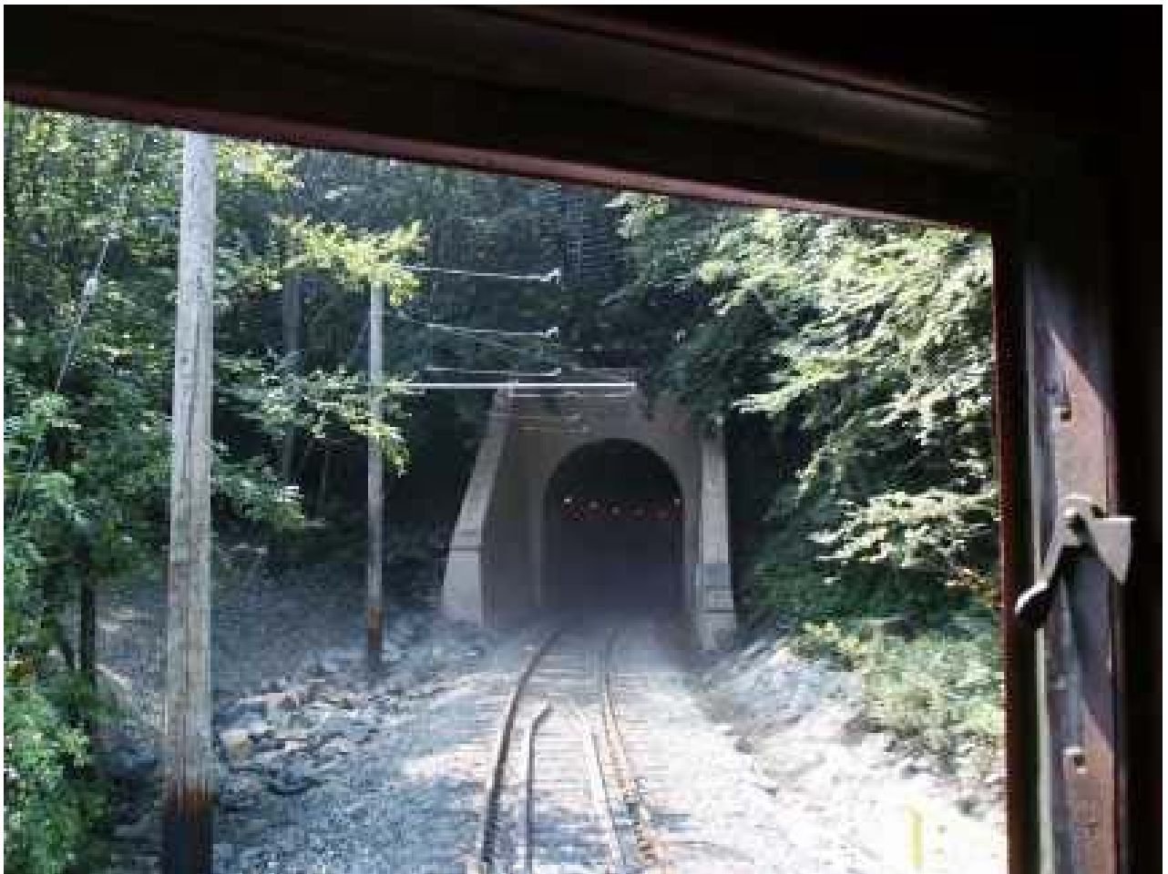
Figure 75: North Portal of Tunnel
