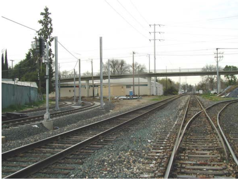
Figure 59: Bee Bridge and Junction with South Line
