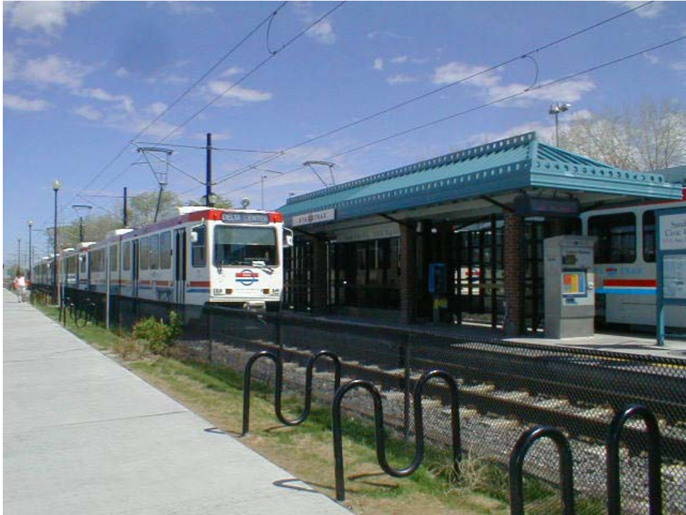
Figure 64: Light Rail Terminal at Sandy, UT
