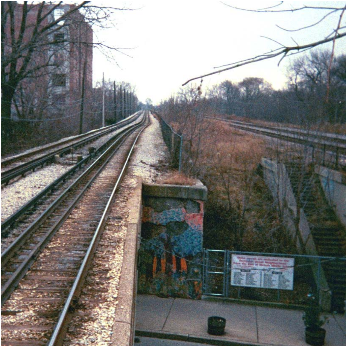
Figure 14: CTA Purple Line at Davis Street, Looking South
