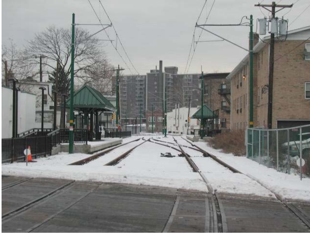
Figure 38: Crossover for Freight Trains at Silver Lake Station
