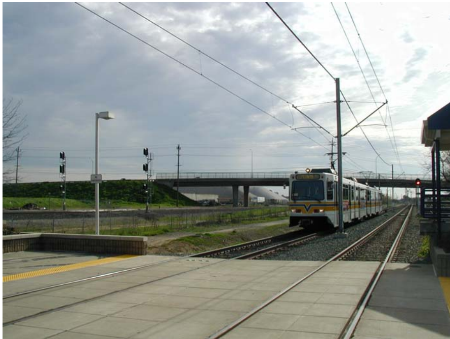
Figure 58: Common Corridor with Union Pacific Railroad at Swanston
