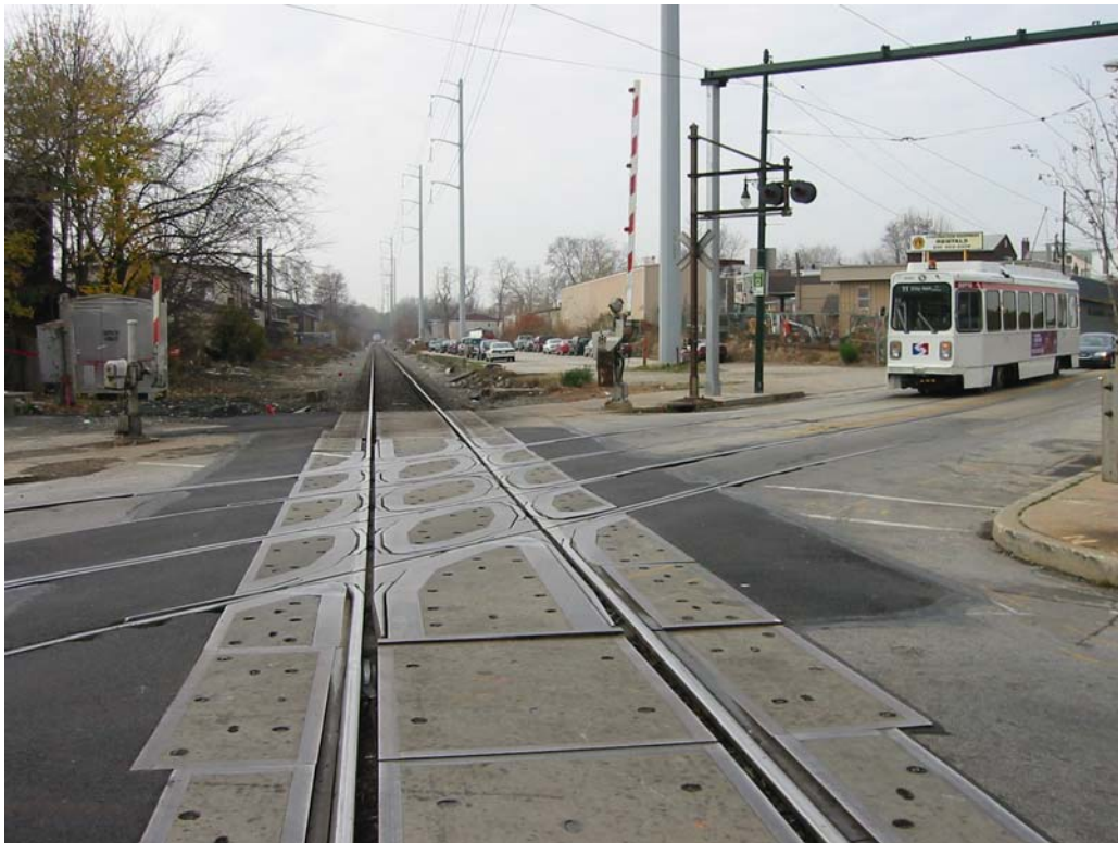
Figure 51: CSXT Grade Crossing with SEPTA Route 11 Trolley, Darby, PA, Looking South
