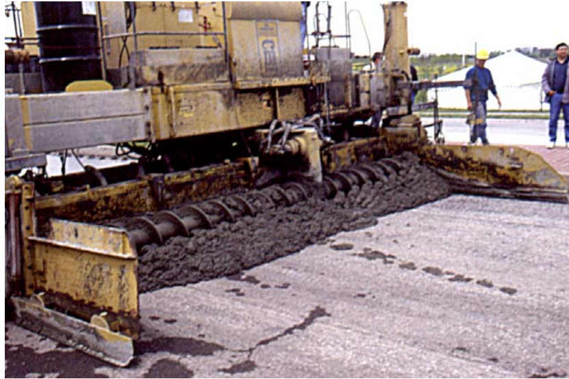
PHOTO 1: Concrete Placement
