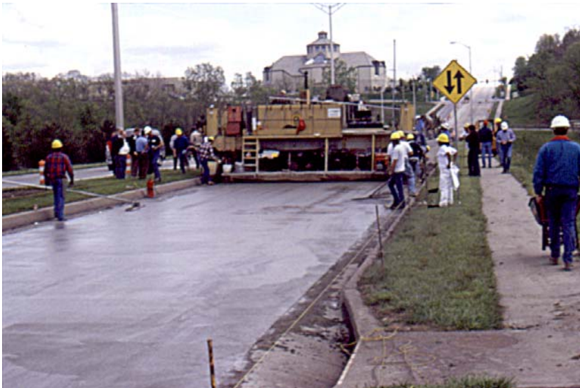
PHOTO 4: Main Line Paving
