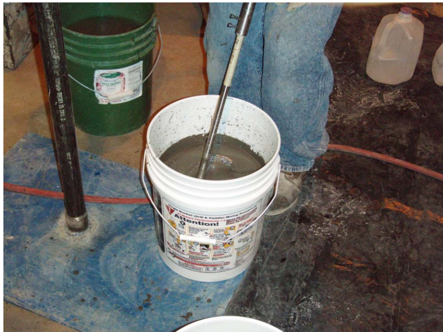
Figure 3-10: Mixing Pavemend 15.0
