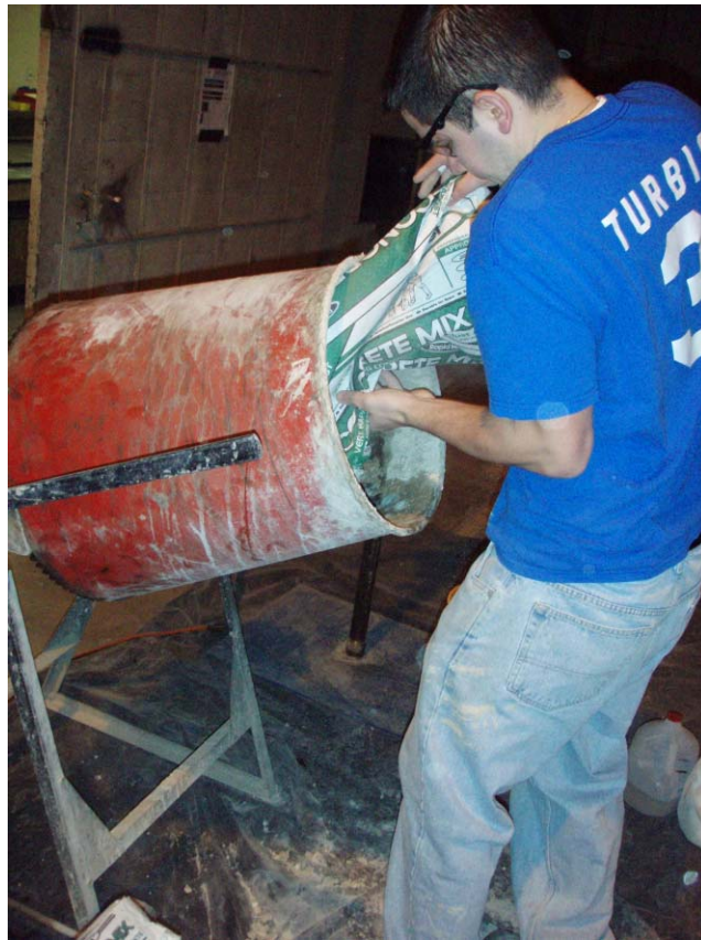
Figure 3-12: Mixing Rapid Set
