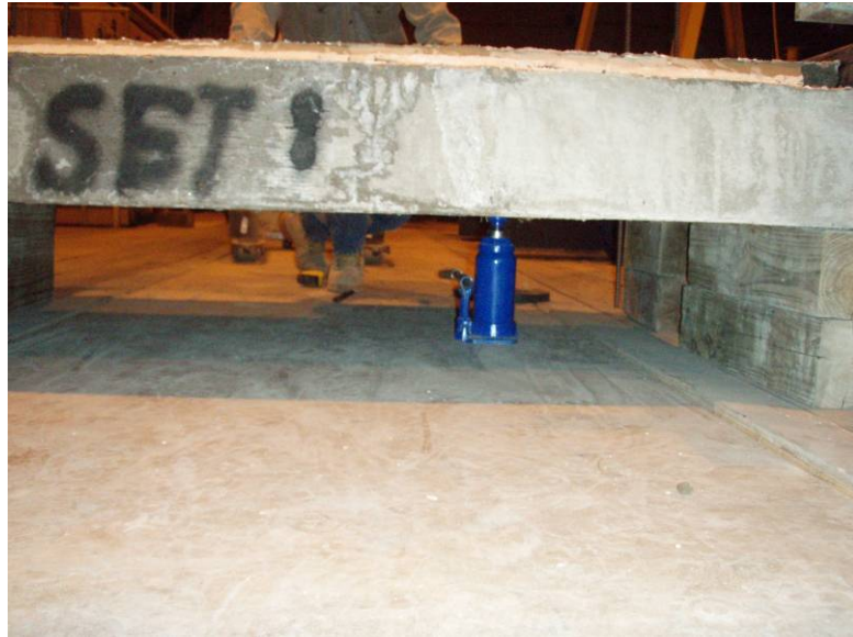
Figure 3-36: Cracking Corrosion Slab – Side View
