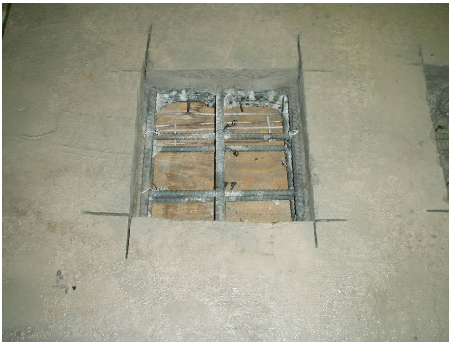
Figure 3-8: Jackhammered Patch Area – Full Depth
