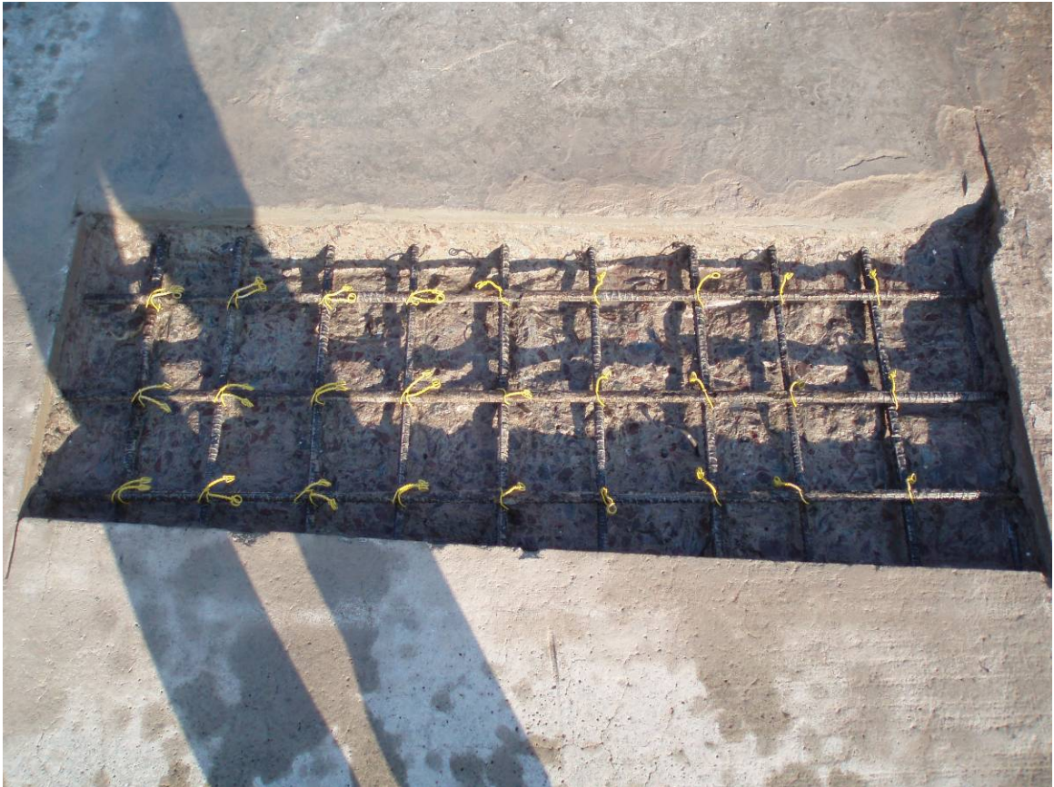
Figure 3-9: Cleaned Patching Hole
