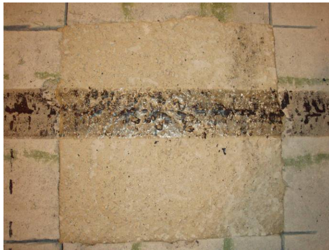
Figure B-12 : Rapid Set Patch after Tire Load Simulation – Close-up 1
