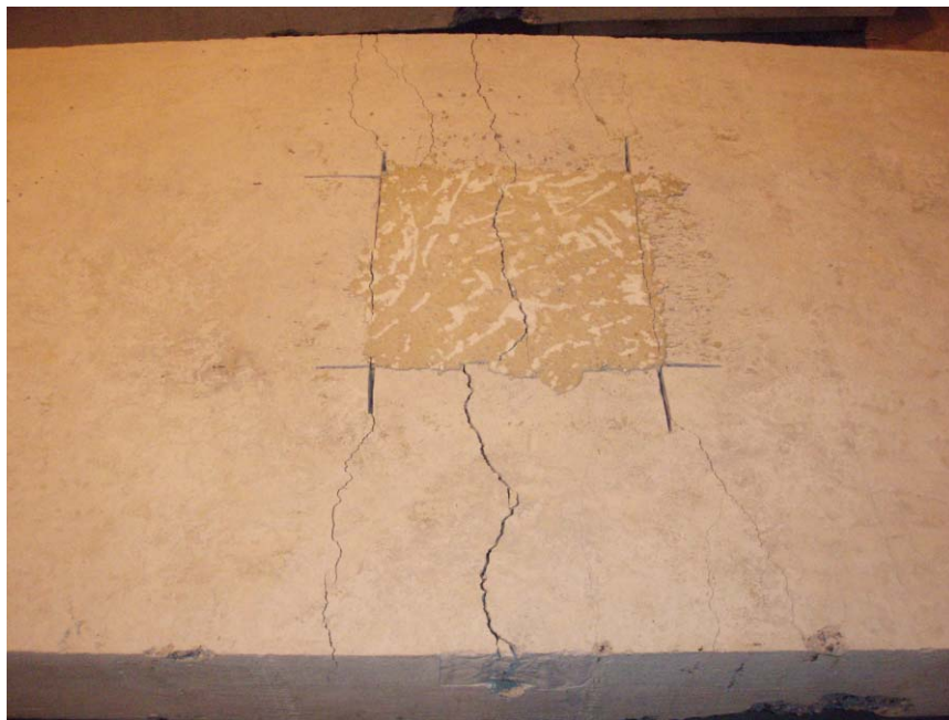
Figure B-6: Three-Point Loading – Rapid Set – Small, Deep
