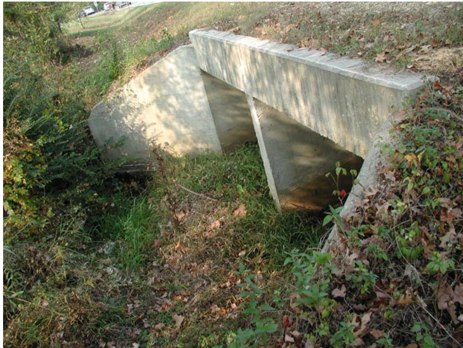
Figure 2-2. Reinforced concrete box culvert
