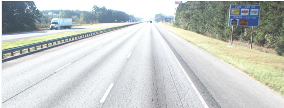
FIGURE I.24: Pavement Conditions of Test Site #11
