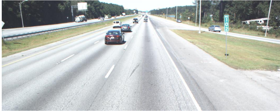
FIGURE I.12: Pavement Conditions of Test Site #2
