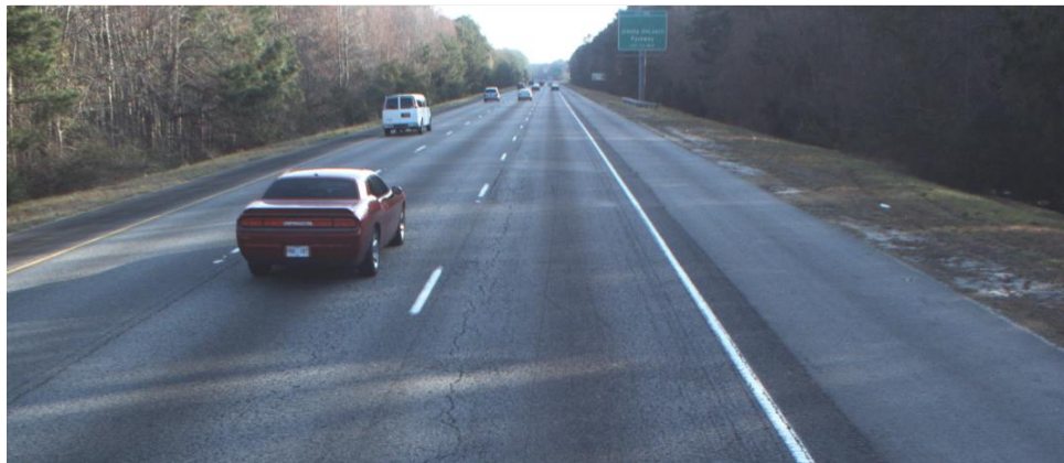
FIGURE I.16: Pavement Conditions of Test Site #4
