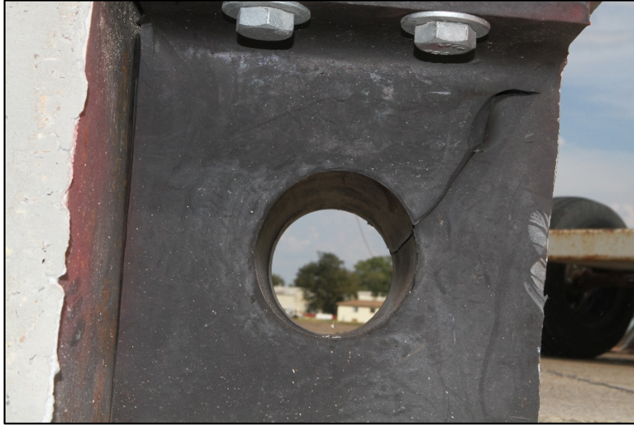
Figure 5.23. Crack in Block after Test No. 468957-B7.
