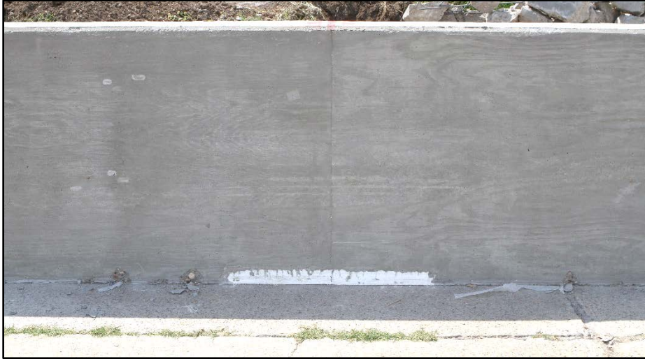
Figure 5.16. Impact Side of Barrier after Test No. 468957-B6.
