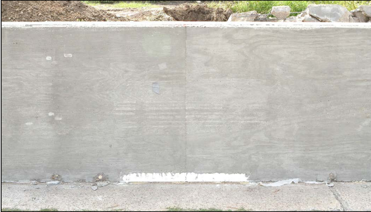
Figure 5.21. Impact Side of Barrier after Test No. 468957-B7.
