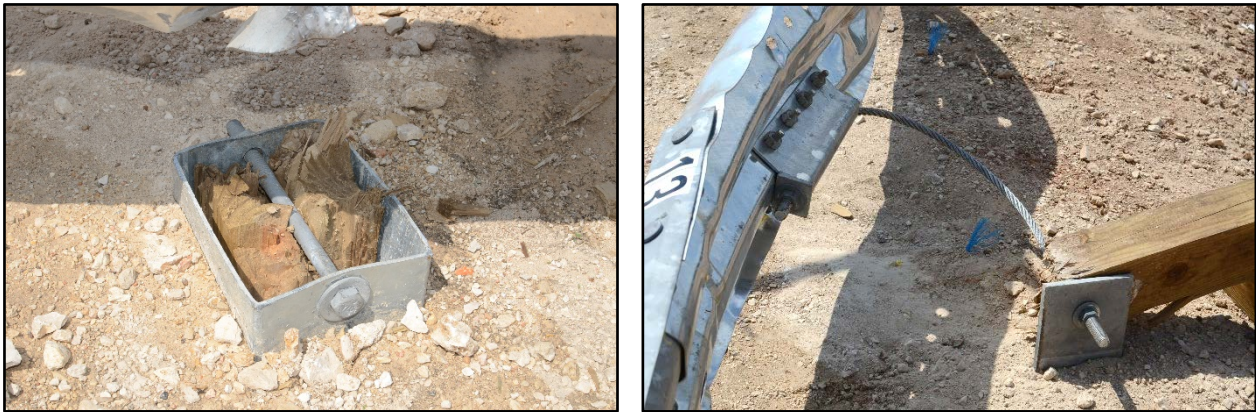
Figure 9.6. Damage to Cable and Post 12 after Test No. 469138-3-3.
