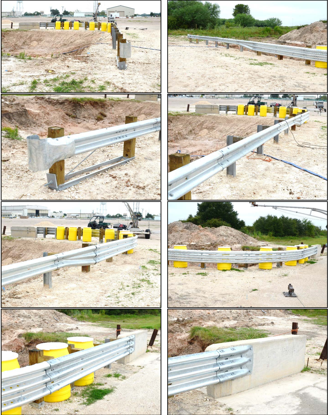
Figure 4.2. TxDOT Low-Speed Short Radius Guardrail Treatment prior to Test Nos. 469137-3-1 and 469138-3-4.
