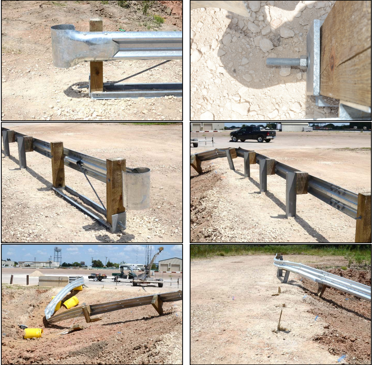
Figure 7.4. Damage to Rail Section Perpendicular to Roadway after Test No. 469137-3-1.
