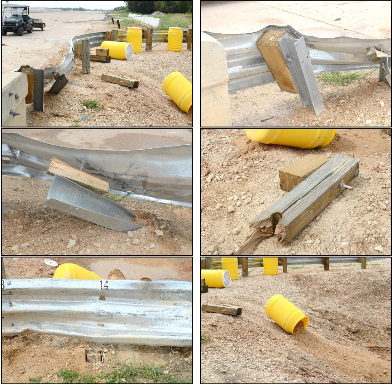
Figure 10.4. Damage to Rail Section Parallel to Roadway after Test No. 469138-3-4.
