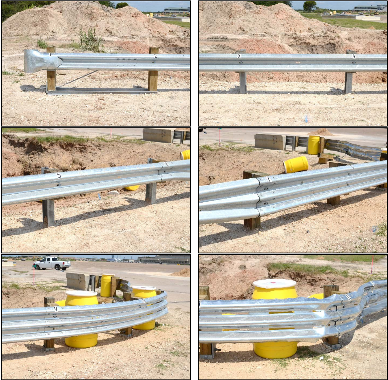
Figure 9.4. Damage to Rail Section Perpendicular to Roadway after Test No. 469138-3-3.
