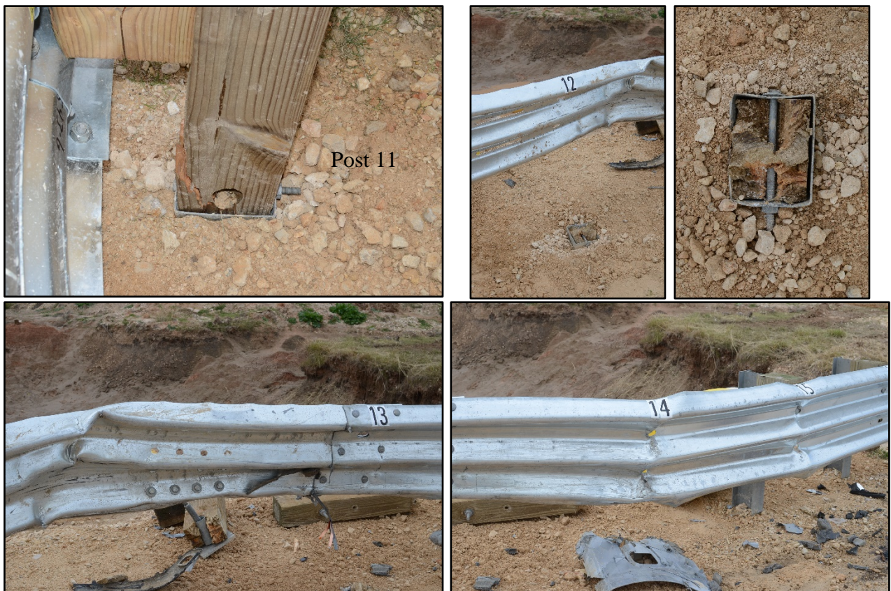
Figure 11.6. Posts 11 through 14 after Test No. 469138-3-5.
