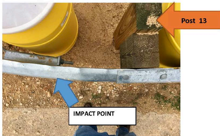
Figure 5.4. Target CIP for MASH Test 2-35 on the TxDOT Low-Speed Short Radius Guardrail Treatment.
