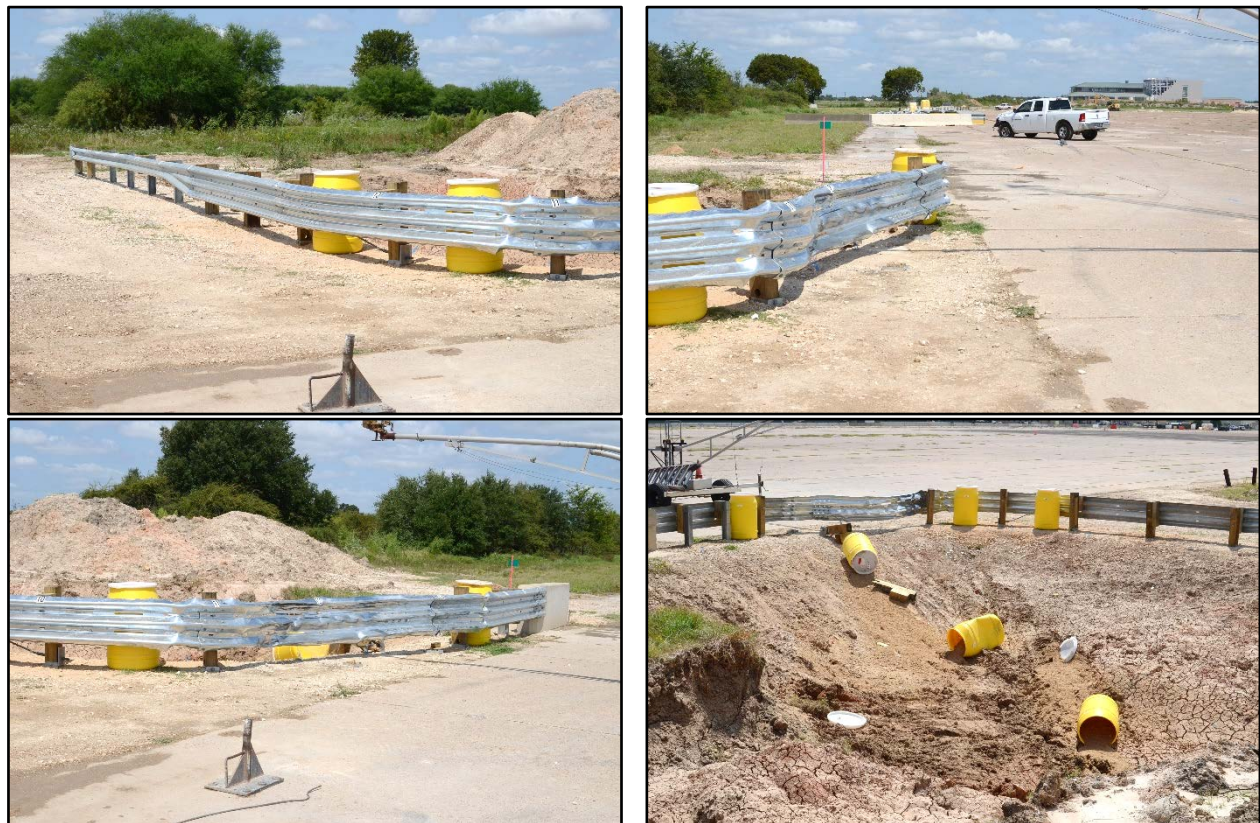
Figure 9.3. TxDOT Low-Speed Short Radius Guardrail Treatment after Test No. 469138-3-3.
