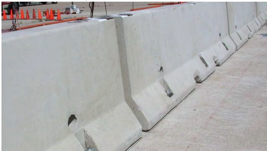
c) Temporary Concrete Barriers with Restrained Movement
