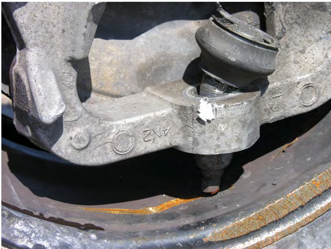
Figure 7. Inside of Wheel Damage, Test No. PCMB-1
