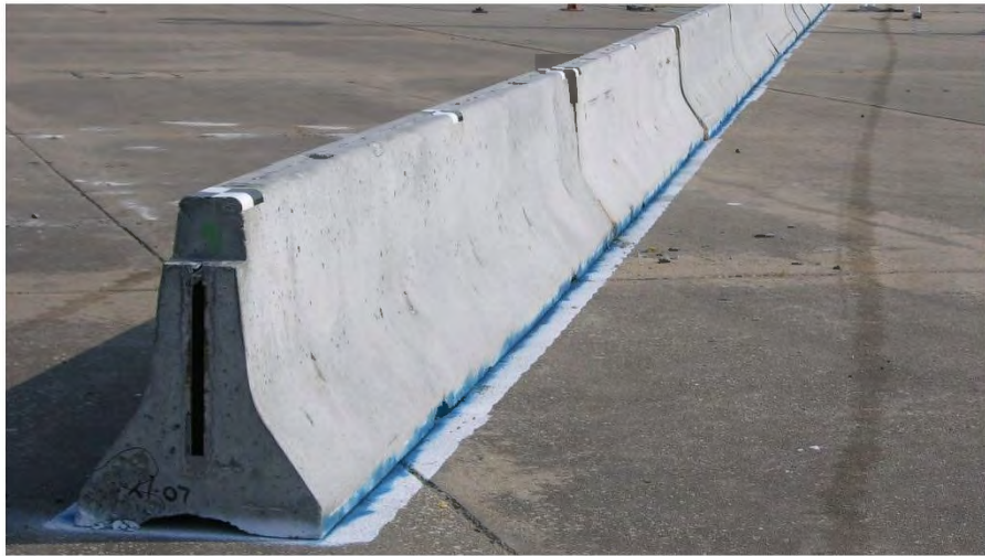
a) Free-Standing Temporary Concrete Barriers
