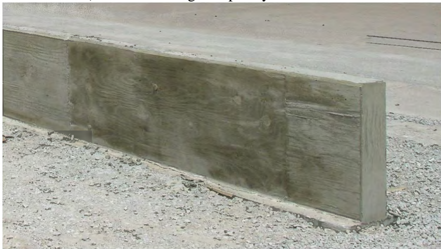
b) Permanent Concrete Barrier
