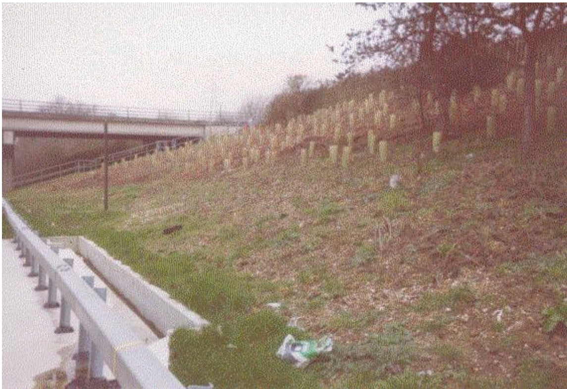
Figure 13.6. Photograph of slope and noise barrier (Site B)
