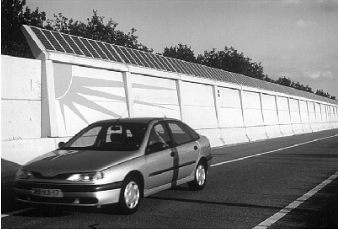
Figure 2.1. Solar panels fitted onto noise barriers (from www.caddet-re.org , by courtesy of CADDET Dutch National Team)
