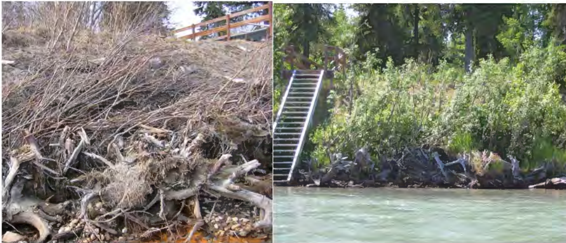
Figure 9. Upper bank brushlayering at Centennial Park. Left photo taken May 2007, right photo taken June 2007.
