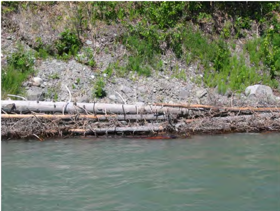
Figure 12. Spruce tree revetment at Soldotna B&B Lodge.
