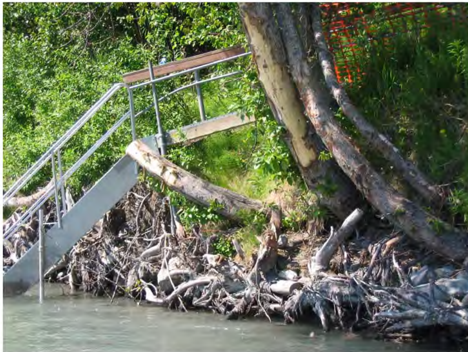
Figure 8. Root wad installation at Soldotna B&B Lodge.
