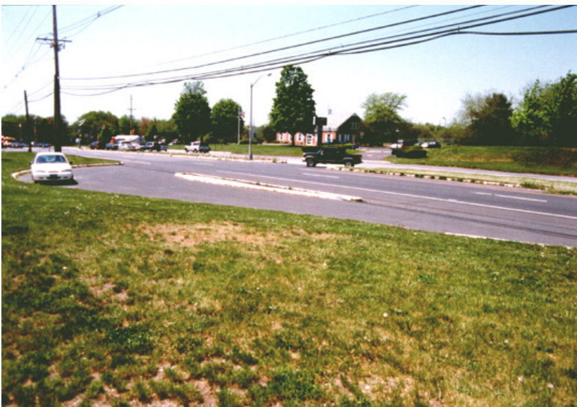
Figure 3. U-turn jughandle facility
