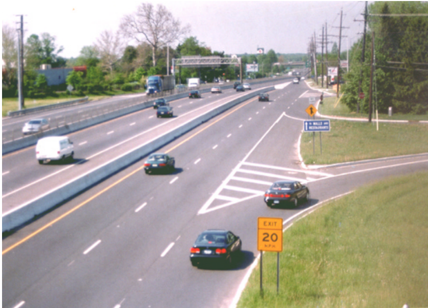
Figure 2. Access management treatments separating driveways from through traffic
