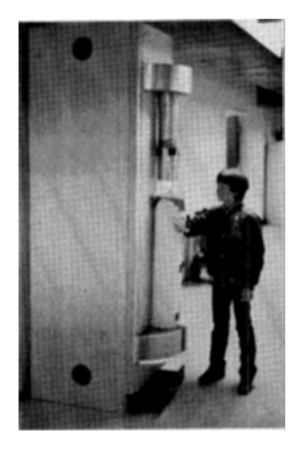
FIG. 11 Air-to-Air Heat Exchanger built from plans developed by Besant [7] at the University of Saskatchewan.
