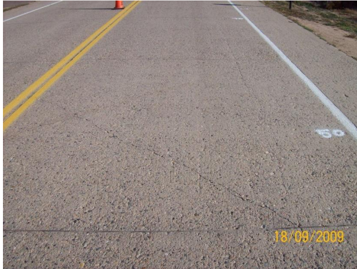
Figure 53. Photo. Transverse (actually diagonal) cracking for trafficked lane for SPS-8 project 0811 in Colorado.
