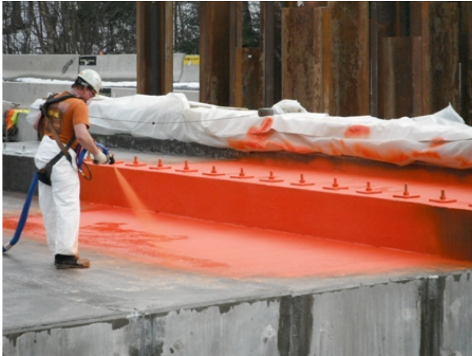
Figure 3: Application of the spray-on membrane (March 12, 2012)
