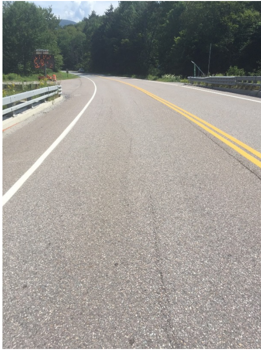
Figure 15: View of bridge overlay, looking south (August 15 ,2017)
