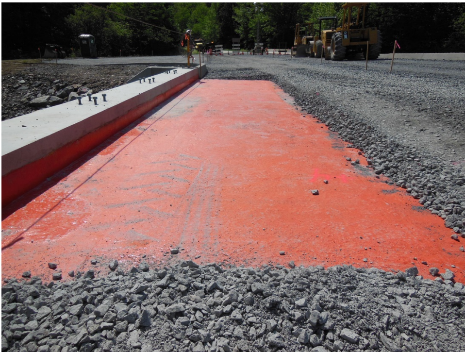
Figure 4: BDM with gravel cover (June 1, 2012)
