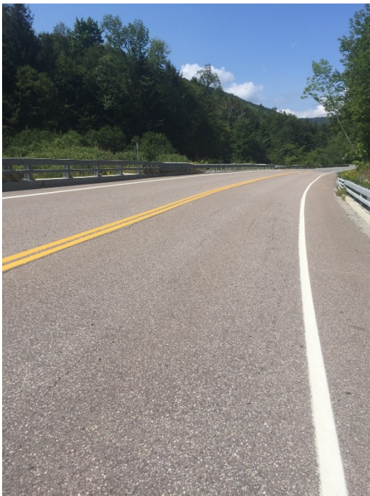
Figure 16: Bridge Overlay, looking north (August 15 ,2017)
