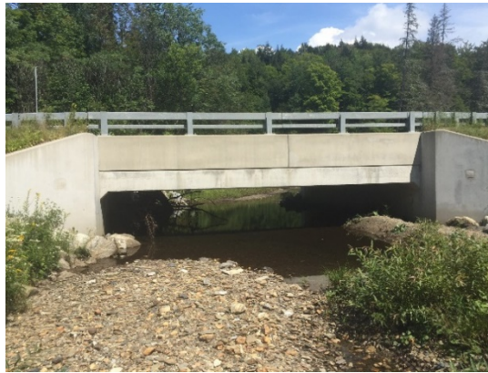
Figure 12: View of Bridge 165 on VT 100 in Warren, right side (August 15 ,2017)
