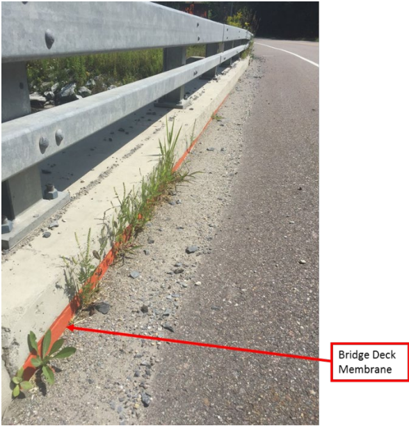
Figure 18: Bridge deck membrane (August 15 ,2017)
