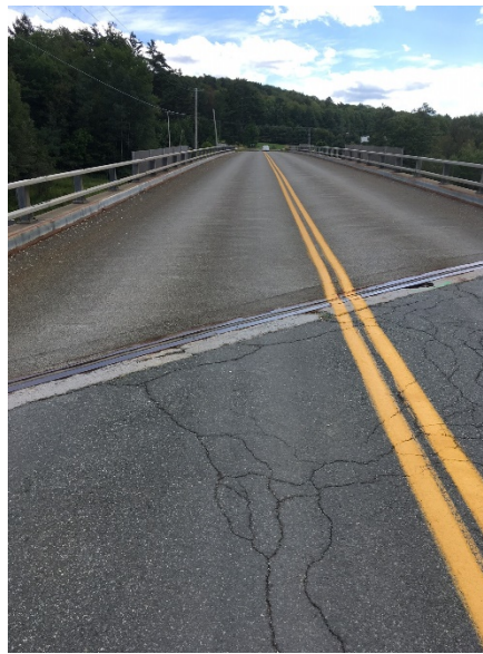
Figure 8: Cracking of southbound approach to bridge 8
