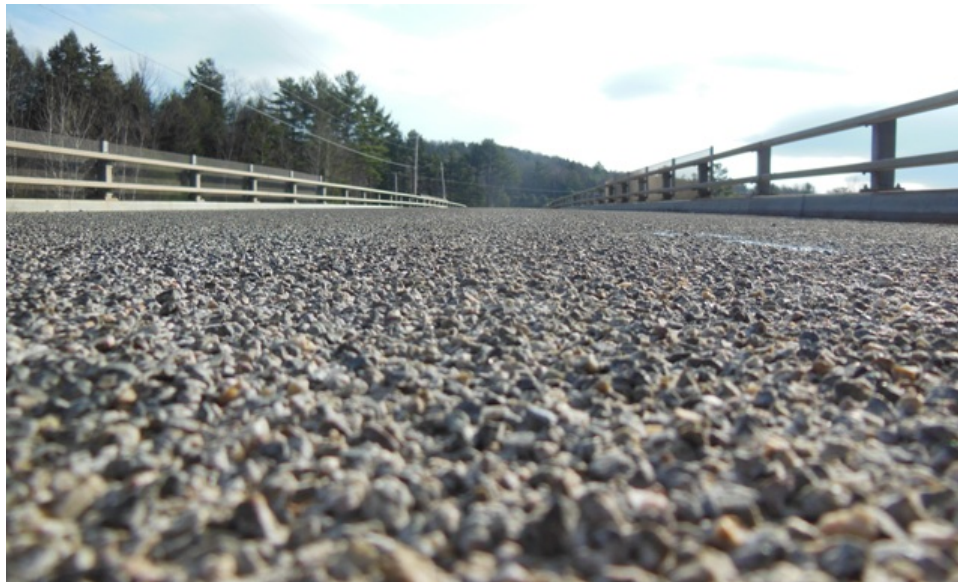
Figure 4: Surface texture of the Flexogrid
