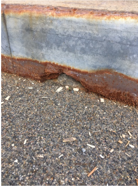
Figure 7: Loose aggregate from Flexogrid surface and rusting of metal curb protector
