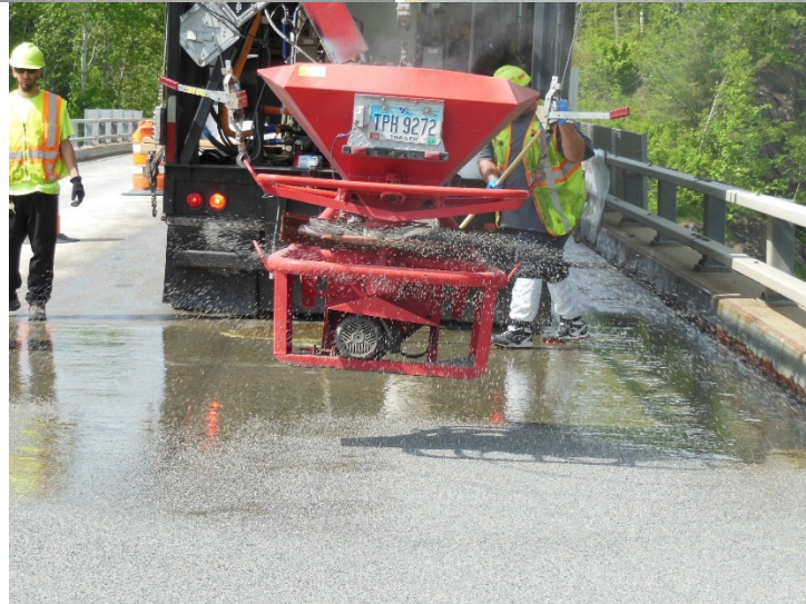
Figure 3: Flexogrid being Applied to the Deck
