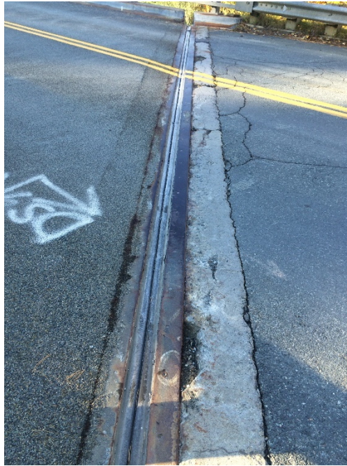
Figure 5: Cracking around bridge joints
