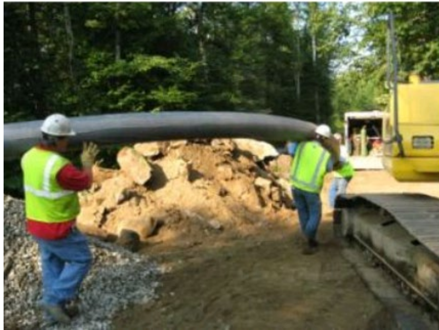
Figure 1: FRP tubes can be carried into place by hand labor (1)
