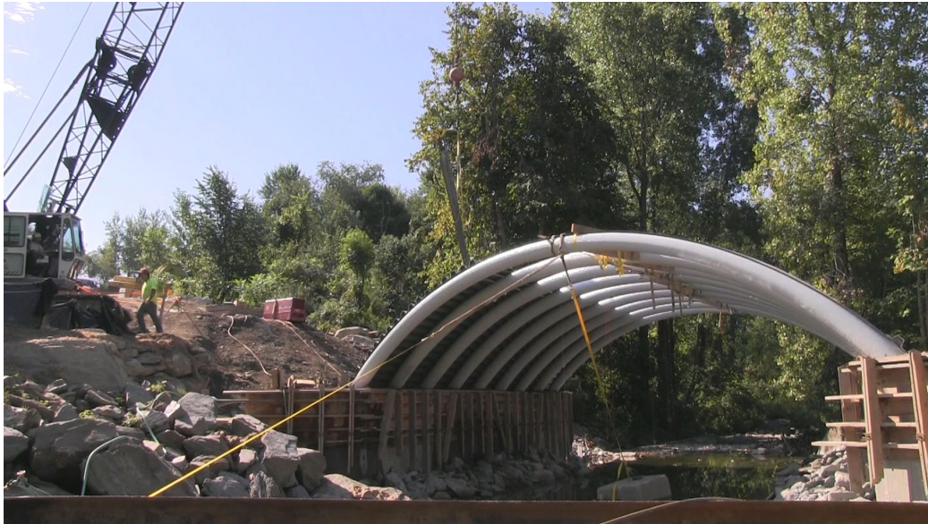
Figure 10: All tubes in place with decking being installed
