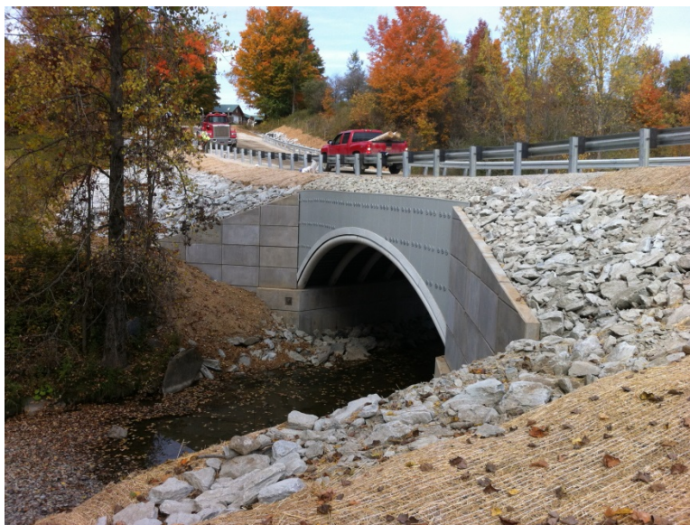
Figure 13: Completed CAB
