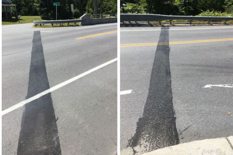
Figure 7: Joints at Bridge 9, appearing to be in good condition
