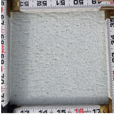
Surface Thermoplastic Utah, Installation, 28-1+00
