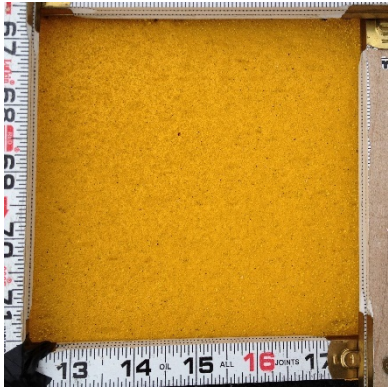
Surface Thermoplastic Utah, Installation, 28-1+00
