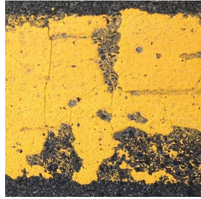
Surface Thermoplastic Wet Reflective, 8 months, 25-4+00
