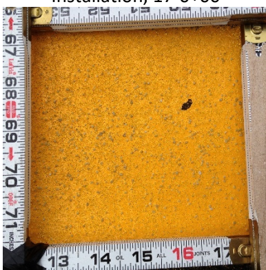
Recess Polyurea Wet Reflective, Installation, 17-0+00
