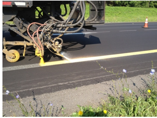
Figure 5: Waterborne binder and optic package being applied.
