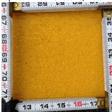
Recess Thermoplastic Wet Reflective, Installation, 23-0+00
