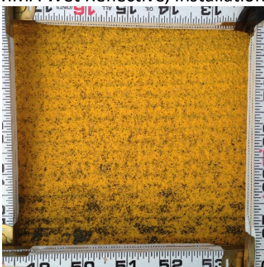
Recess MMA Wet Reflective, Installation, 7-0+00
