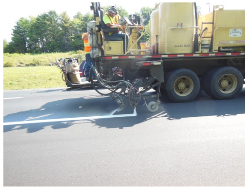
Figure 6: White waterborne binder and optic package being applied.
