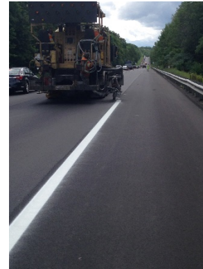
Figure 10: Polyurea binder being applied by the truck.
