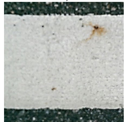
Recess Epoxy Utah, 36 months, 35-0+00
