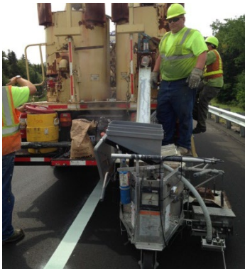
Figure 7: Thermoplastic cart being filled at the truck.
