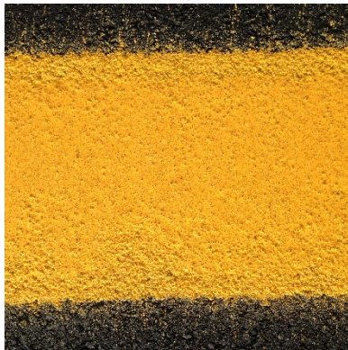
Surface Epoxy Utah, Installation, 29-0+00
