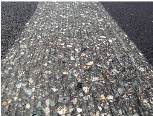
Figure 3: Recessed pavement section for marking application
