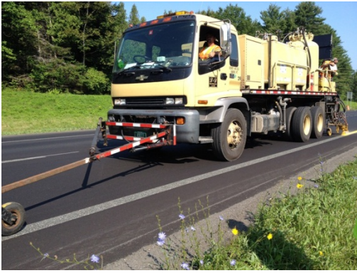
Figure 4: Applying the yellow waterborne stripe.
