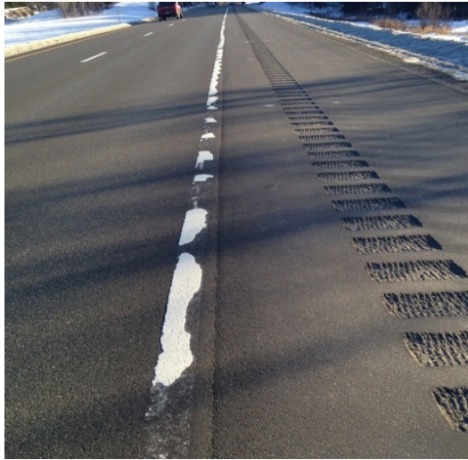
Figure 25: TS 28 Damage Overview
