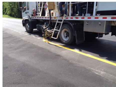
Figure 14: Optic package and paint being applied.
