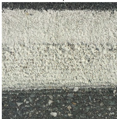
Recess Polyurea Wet Reflective, 15 months, 17-0+00
