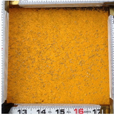
Surface Polyurea Wet Reflective, Installation, 15-0+00
