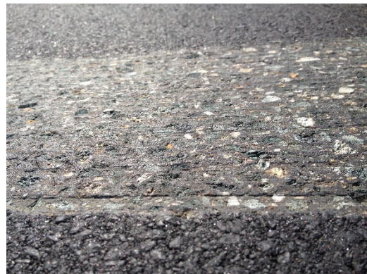
Figure 3: Recessed pavement section for marking application
