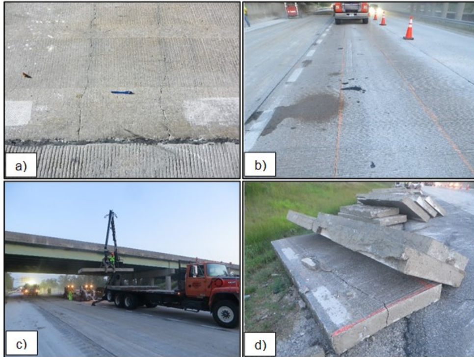
Figure 12. Patching on SR 288: a) area to be patched with closely spaced cracks; b) area selected for patching; c) old concrete slabs being removed; d) removed concrete slabs
