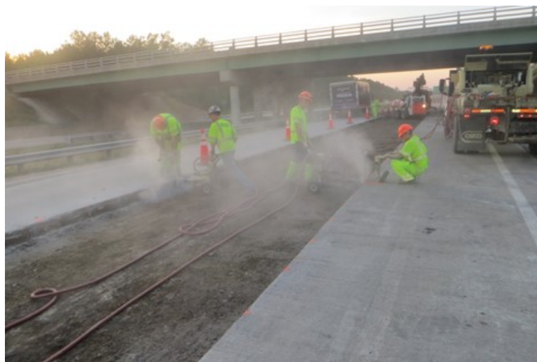
Figure 13. Longer of Two Patches on SR 288 Constructed on 6/10/14
