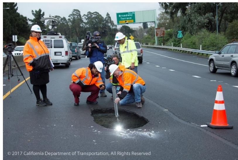
FIGURE 2: SINKHOLE ON HIGHWAY 13
