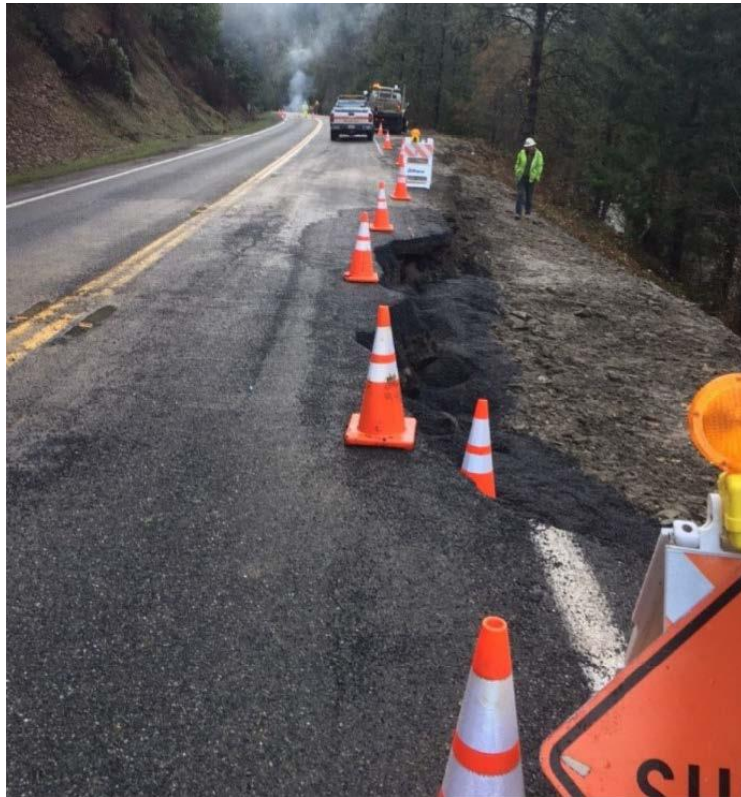
FIGURE 6: EROSION ON SR 96 NORTH OF SOMES BAR
