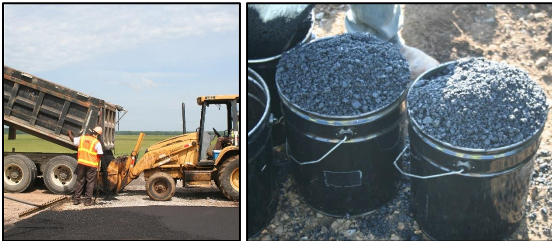
Figure 2.5. CAFB Material Sampling
